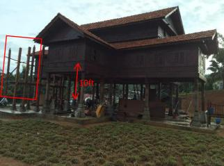
Figure 8: Original condition before (dismantle-left) and after (reassembled-right) where the height of underneath was increased to 10ft, features of dragon head at the end of roof ridge was not constructed (red circle)and new staircase (red rectangle)Source: Sulaiman (2017)
