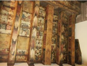
Fig. 4 – 302/4 Lawnmarket 2010 restoration; Fig. 5 – Gladstone's Land 1980s restoration; plaster over 'plastic-wood remains'. plaster fills, neutral tone stippling.
