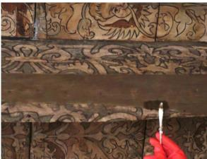
Fig. 6 – Riddle's Court 1960s restoration; cable holes cut in 16thC boards.
