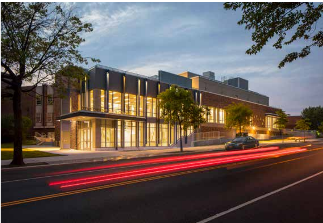
Susan E. Wagner High School Performing Arts Center Staten Island, NY
