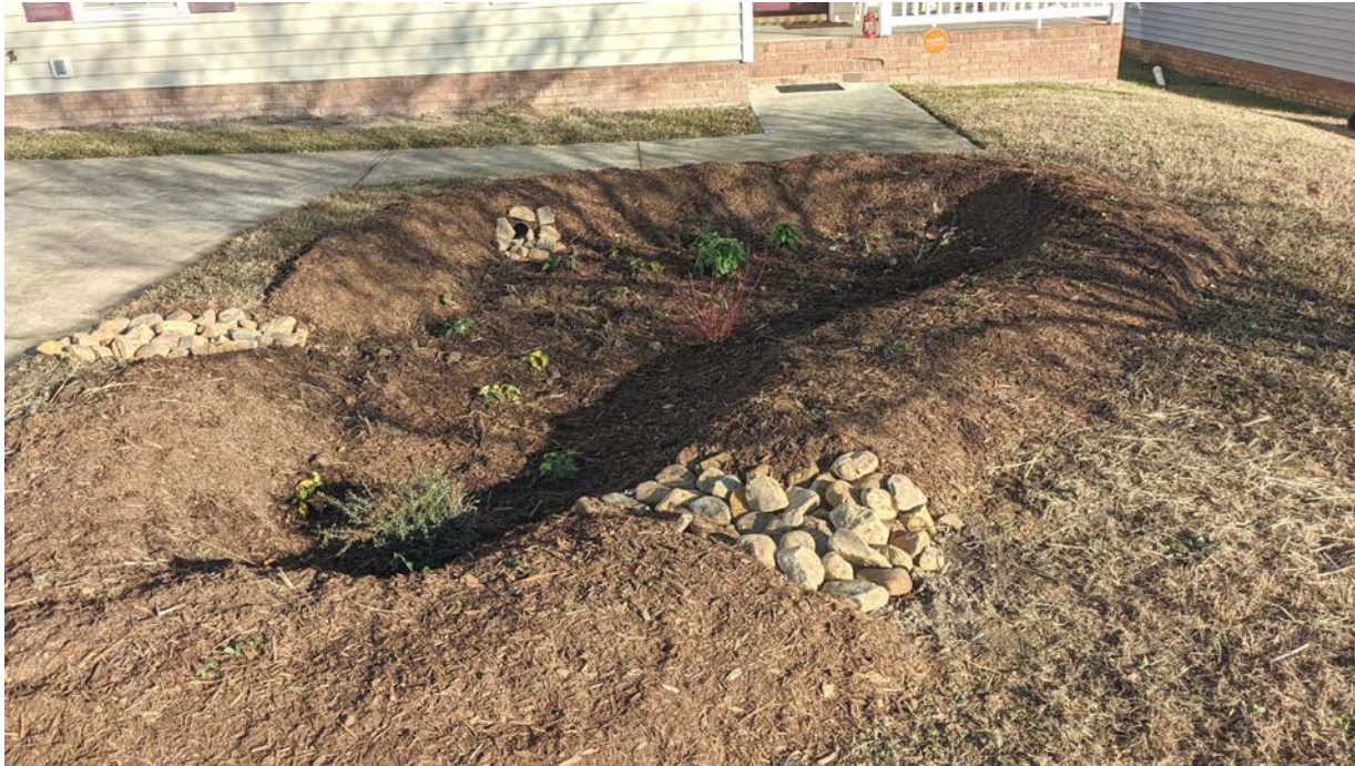
Completed rain garden at 808 Elkhart Dr.
