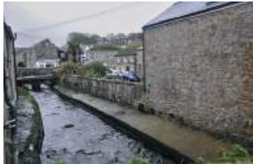
Fig. 6 Above. Old Tolcarne Bridge, Newlyn Henry Pendarves Tremenheere 1804. (image courtesy of Penlee House Gallery and Museum, Penzance) Below. Today, the Old Tolcarne Bridge is now squeezed by development and prone to flooding. (November 2020 MAT)
