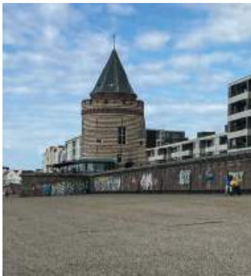
Fig. 19 Vlissingen. The remaining city tower on the sea wall. The other half was damaged by storm action and was demolished.
