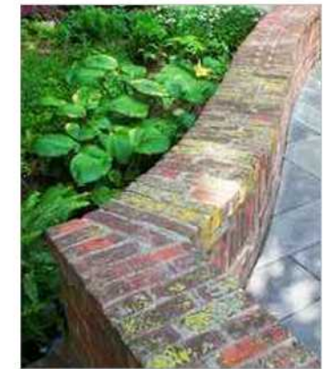
Curved brick wall / seat
