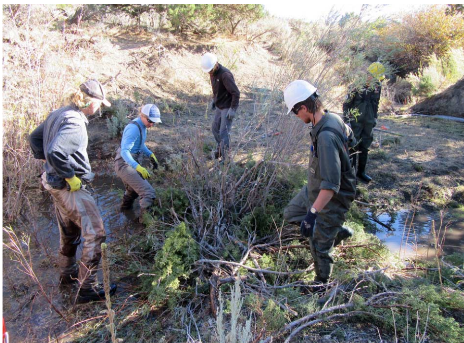
From left: Construction of one BDA (Beaver Dam Analogue) during a restoration project in Northern Utah rangelands... and another BDA one year after construction.
