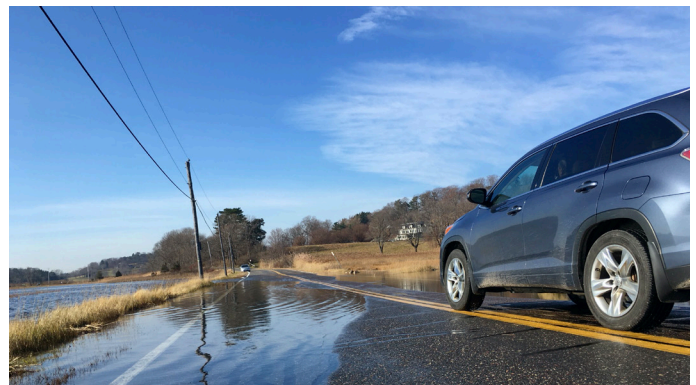
Argilla Road flooding
