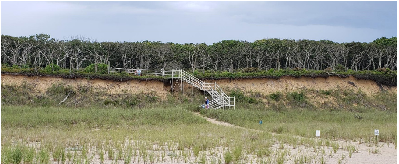
Portable modular aluminum stairs can be removed before major storms. Stairs allow safe visitor access without eroding the banks. Photo credit: Tom O'Shea
