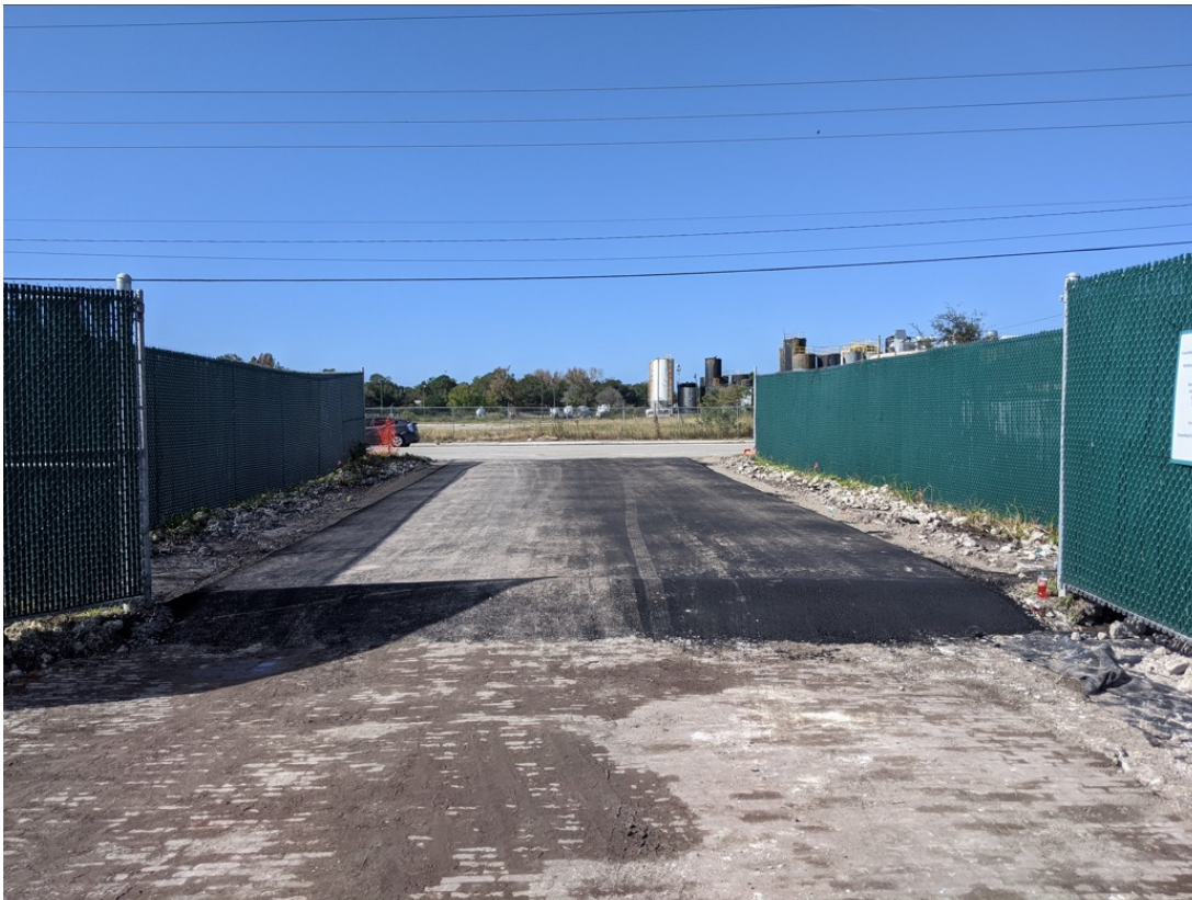
Asphalt entrance road
