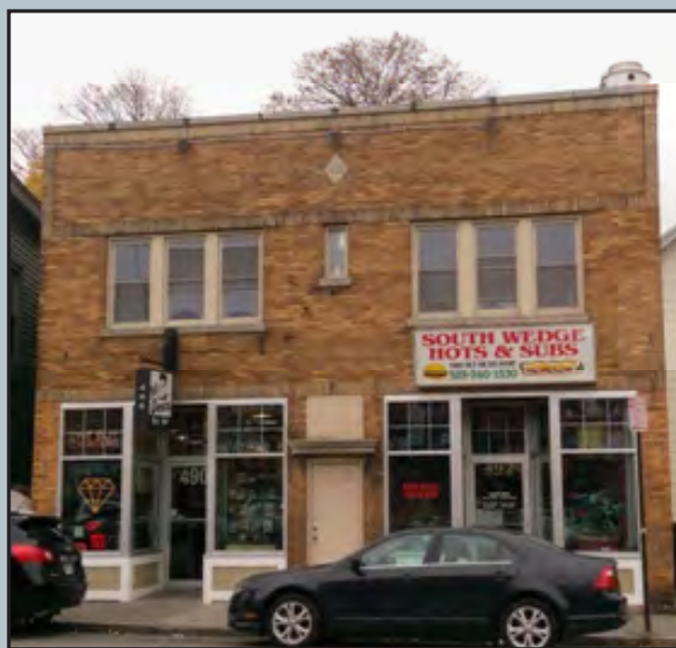
490 Monroe Ave. before renovation. (Photo - Brody Real Estate LLC)
