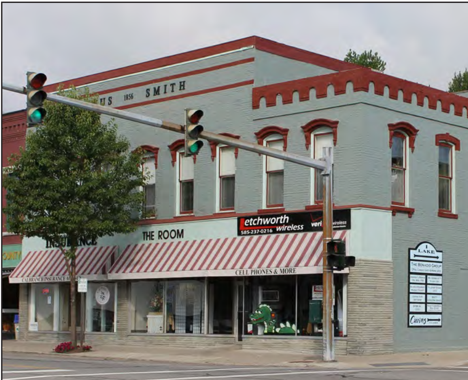
Rufus Smith Building. In 2008 the Rufus Smith block in downtown Perry underwent $700,000 dollars in renovations thanks to the Perry New York LLC (PNY).
