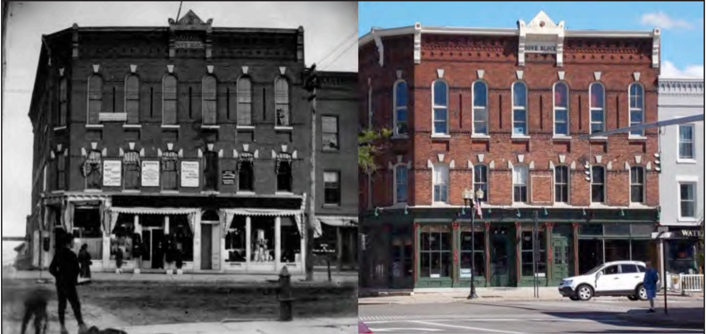
Historic and present day photos of the Dove Block, 459-465 Exchange Street. (Photo - Johnson-Schmidt & Associates)
