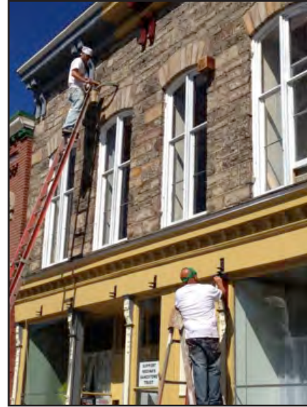
Exterior Rehab work on 409-413 Main St. Medina, 2014. (Photo - Christopher Busch)
