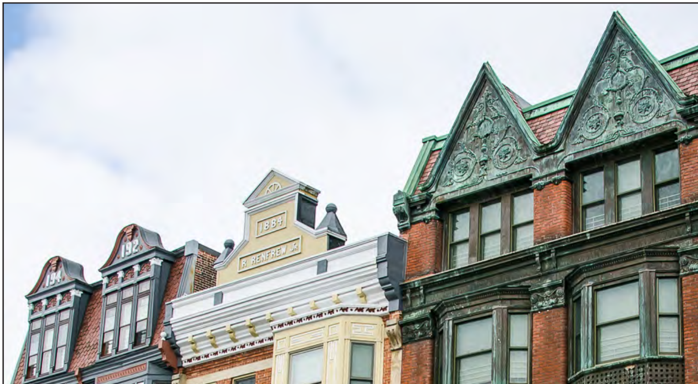
Frederick Douglass Apartments. Historic tax credits were used for the building renovations. See Case Study – A Rochester Urban Row Success Story for more information. (Photo - Suzanne Neace Photography)
