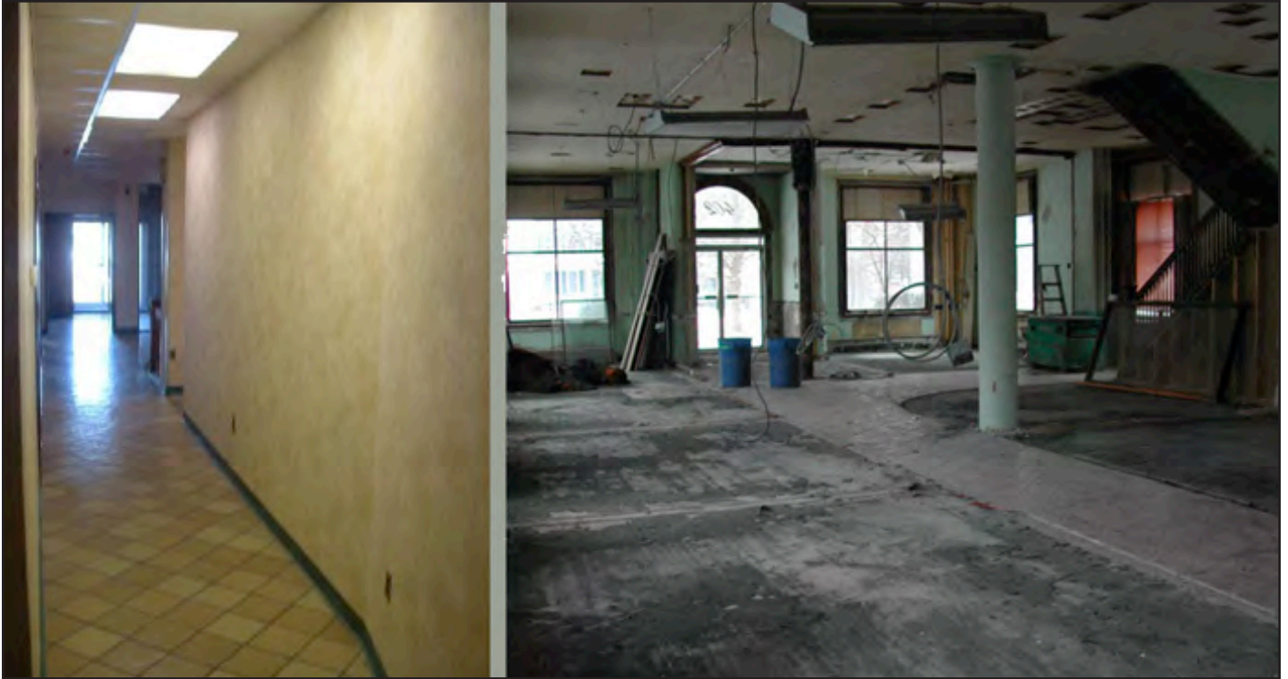
At left, the first floor subdivided into multiple rooms. At right the first floor space after demolition of non-historic partitions. (Photos - Bero Architecture, PLLC)
