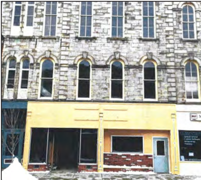
409-413 Main St. Medina, pre-renovation. (Photo - Christopher Busch)
