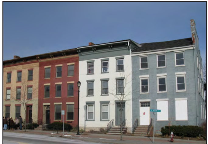
Row houses on East Main Street in the Village of Palmyra’s downtown. (Photo - G/FLRPC)
