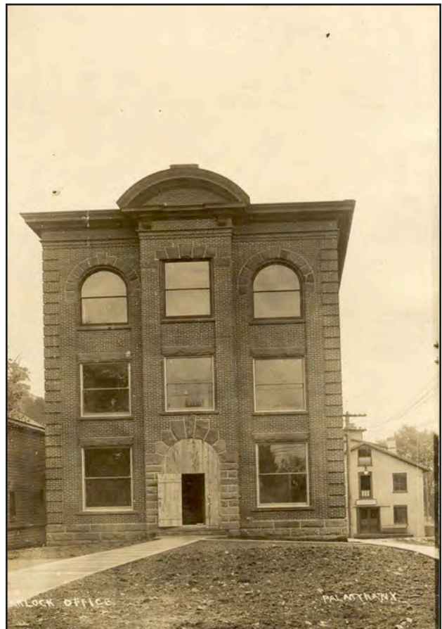
The Garlock Office Building during construction, c.1907. (Photo - Palmyra Community Library)
