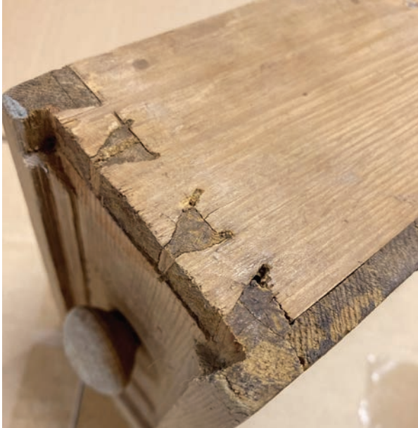
Fig. 6 In this cupboard of vernacular origin the inner cuts of the dovetail joints have been made with drill and a thin sawblade. Nordiska museet. Photo Johan Knutsson.
