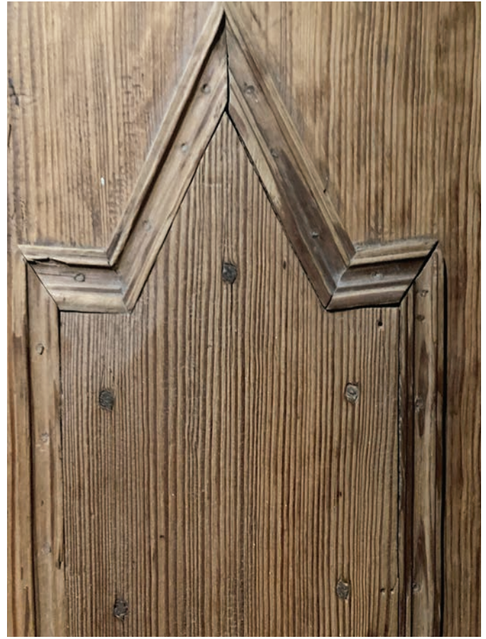
Fig. 3 Obviously the craftsman behind this vernacular cupboard from the 18th century considered it more important to keep the joining of the molding parts together than to achieve a perfectly regular shape of the framing outline. Sörmlands museum. Photo Johan Knutsson.
