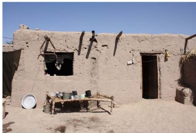
SHELTER PROVIDED AT A KILN IN SURKHROAD
