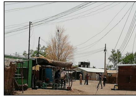
Photo 6 - Electricity available in the market area only
