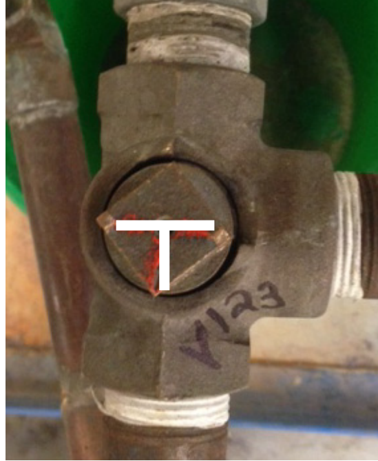
Figure 25. Three-way valve V-123 allowing steam out of Hair Pin HX
