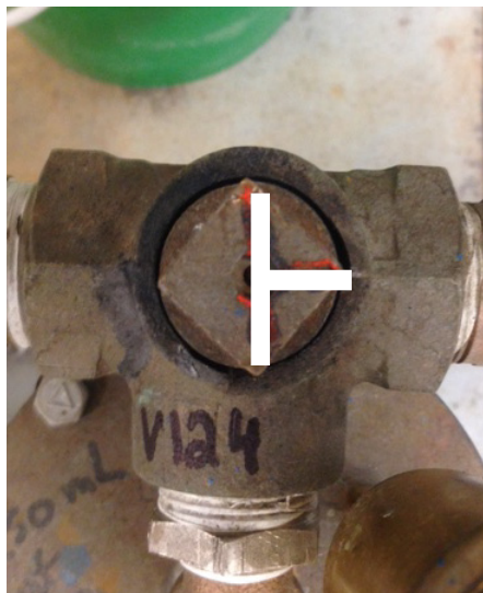
Figure 26. Three-way valve V-124 to condensate trap
