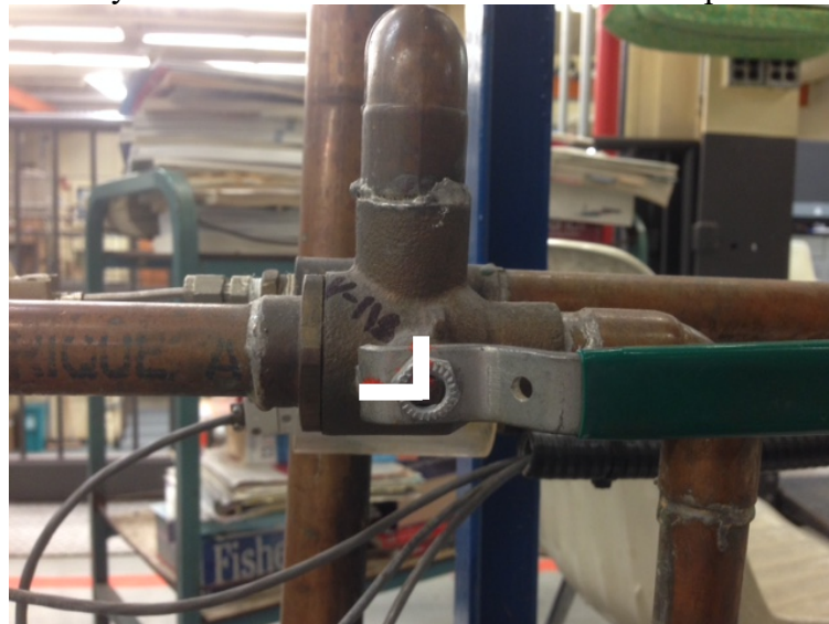
Figure 8. “Three-way valve” V-118 for condensate return
