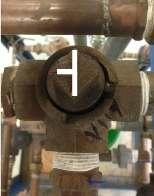
Figure 24. Three-way valve V-119 introducing steam to Hair Pin HX
