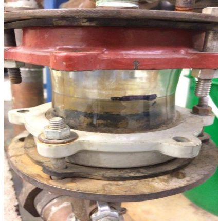
Figure 28. Single and plate HX condensate trap
