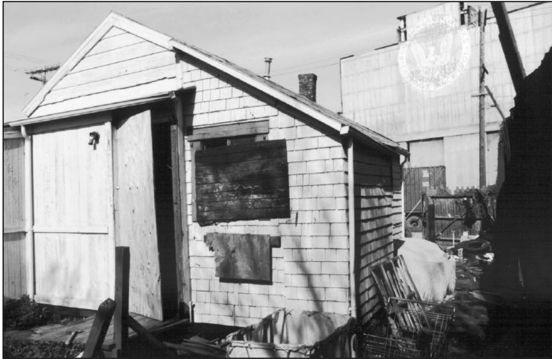
PLATE 28. REAR VIEW OF ADDITIONS AT THE CROWLEY COTTAGE, 1825 SHOREY STREET. This view shows the very informal final addition made to the back of the cottage after World War II. Phoenix Iron Works is visible in the rear of the picture. (Credit: Paul Groth)
