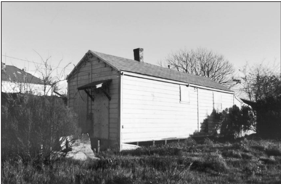
PLATE 27. SIDE VIEW OF THE CROWLEY COTTAGE, 1825 SHOREY STREET. The original two-room house probably ended just beyond the small window on the side elevation, near the vertical trim piece. The chimney roughly indicates the center of the initial building. (Credit: Benjamin Chuaqui)
