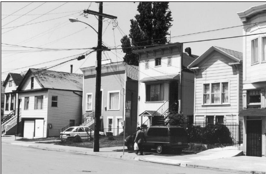
PLATE 14. VARIED SETBACKS ALONG FIFTH STREET, NEAR CHESTER STREET. The variety of different front-yard sizes seemed “strangely varying” to visitors from more expensive neighborhoods. Former front yards convert well to parking spaces. (Credit: Paul Groth)
