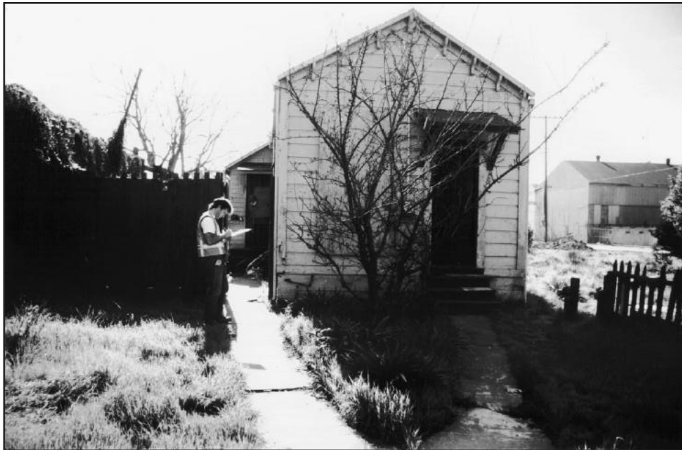
PLATE 26. FRONT VIEW OF THE CROWLEY COTTAGE, 1825 SHOREY STREET. The small scale of the original cottage, constructed in 1874-1875, is apparent, as are the generous front and side yards. Modest brackets decorate the front facade. (Credit: Paul Groth)
