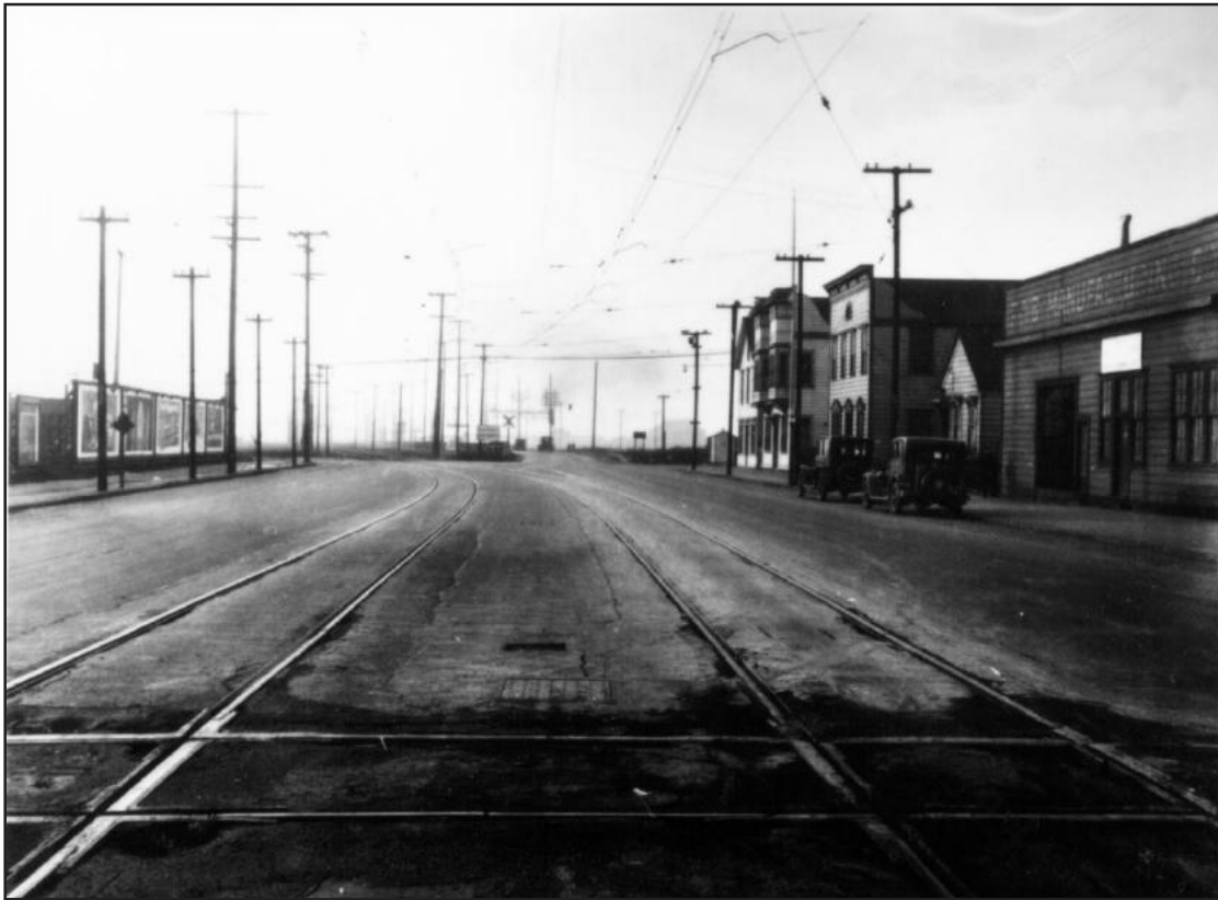
PLATE 8. THE RAILROAD EXCHANGE HOTEL AND OTHER BOARDING HOUSES WEST OF CEDAR STREET IN 1925. The peaked roof of the Railroad Exchange Hotel, built in 1864, is almost obscured by the double-bay windows of an additional rooming house added to the complex in 1890. The Railroad Exchange Hotel, which was the earliest and most enduring boarding house within the project area, yielded significant archaeological deposits representing the hotel's railroad employee tenants. (From the collection of Vernon J. Sappers.)
