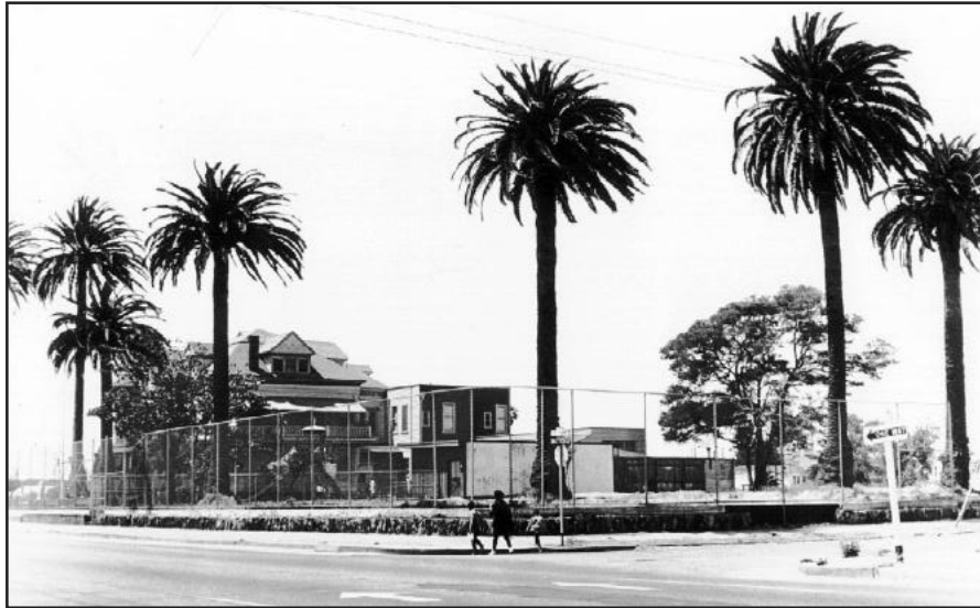
PLATE 66. St. VINCENT'S DAY HOME, 1086 EIGHTH STREET, mid-1960s. In the early 1960s the Oakland Redevelopment Agency accrued a great deal of property adjacent to St. Vincent's in preparation for a very large slum-clearance project. St. Vincent's managed to survive and stands in this picture as the lone survivor of a once-vibrant urban landscape. The Acorn Public Housing Project now surrounds the establishment. (Photo courtesy of the St. Vincent's Day Home)
