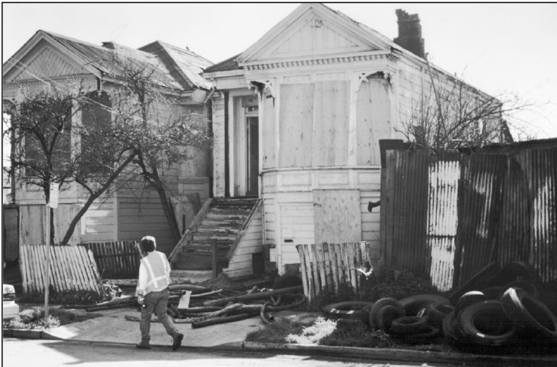
PLATE 21. FRONT VIEW OF THE STEPHENS/WOOD HOUSE, 1817 SHOREY STREET. The facade of the house matches polite styles that could be found in much more expensive neighborhoods. In this view, windows are covered in preparation for moving the house. (Credit: Paul Groth)
