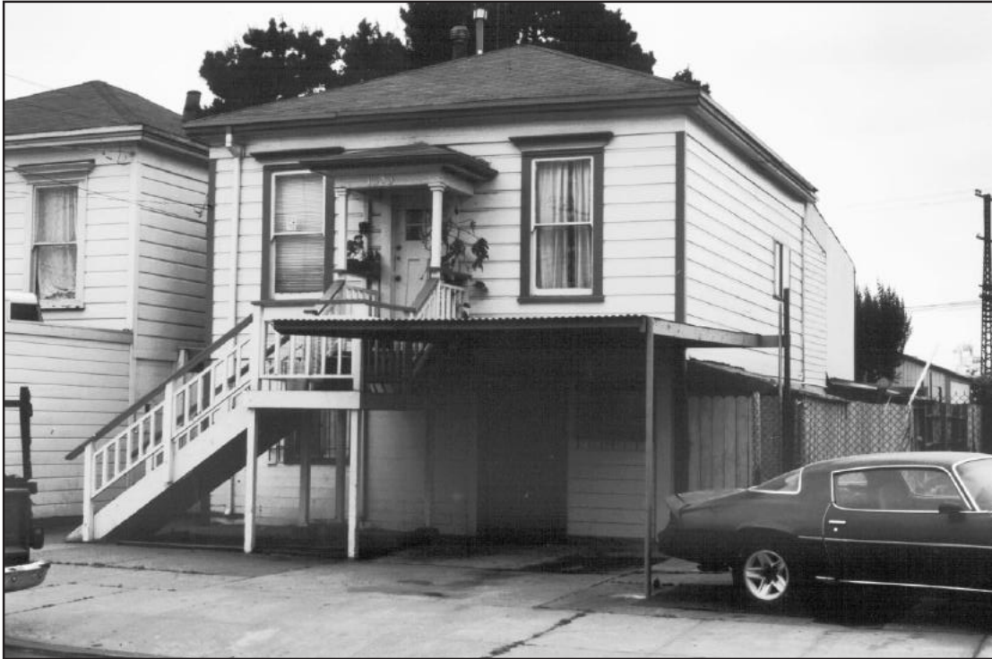
PLATE 32. SIDE VIEW OF THE PORTER/JOST COTTAGE AT 1529 THIRD STREET. The original building is under the hipped roof (and outlined in dark trim boards). Two subsequent rear additions are visible along the side, indicated by the different kinds of siding. The car port, the stair to upper unit, and the sheds in side and rear yard are other recent changes to the building. (Credit: Paul Groth)
