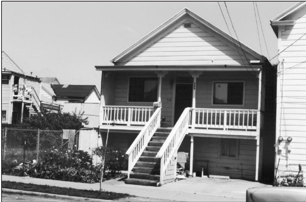
PLATE 29. FRONT VIEW OF SUGRUE/CROSSMAN COTTAGE, 360 CHESTER STREET. The front porch, stairs, and possibly the raised basement are later additions to the 1874-1875 cottage. The side yard to the left informally encroaches on adjacent property, left empty after the neighboring house burned a few years ago. (Credit: Paul Groth)
