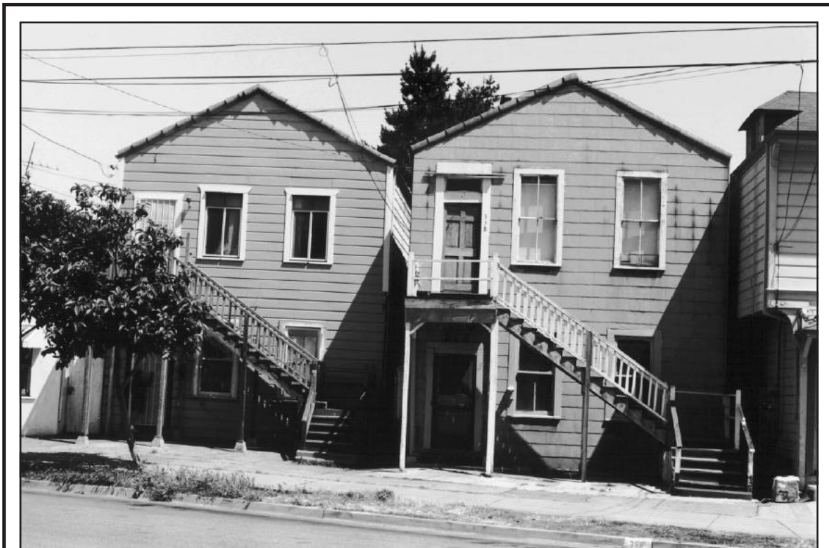
PLATE 38. FRONT VIEW OF THE DAVIDSON/PATTERSON FLATS, 362-364 PERALTA STREET. These two small speculative houses, constructed by James Davidson in the late 1870s, were built as identical one-story, wood-framed buildings. Between 1902 and 1912, they were raised and converted into two-story flats. (Credit: Paul Groth)
