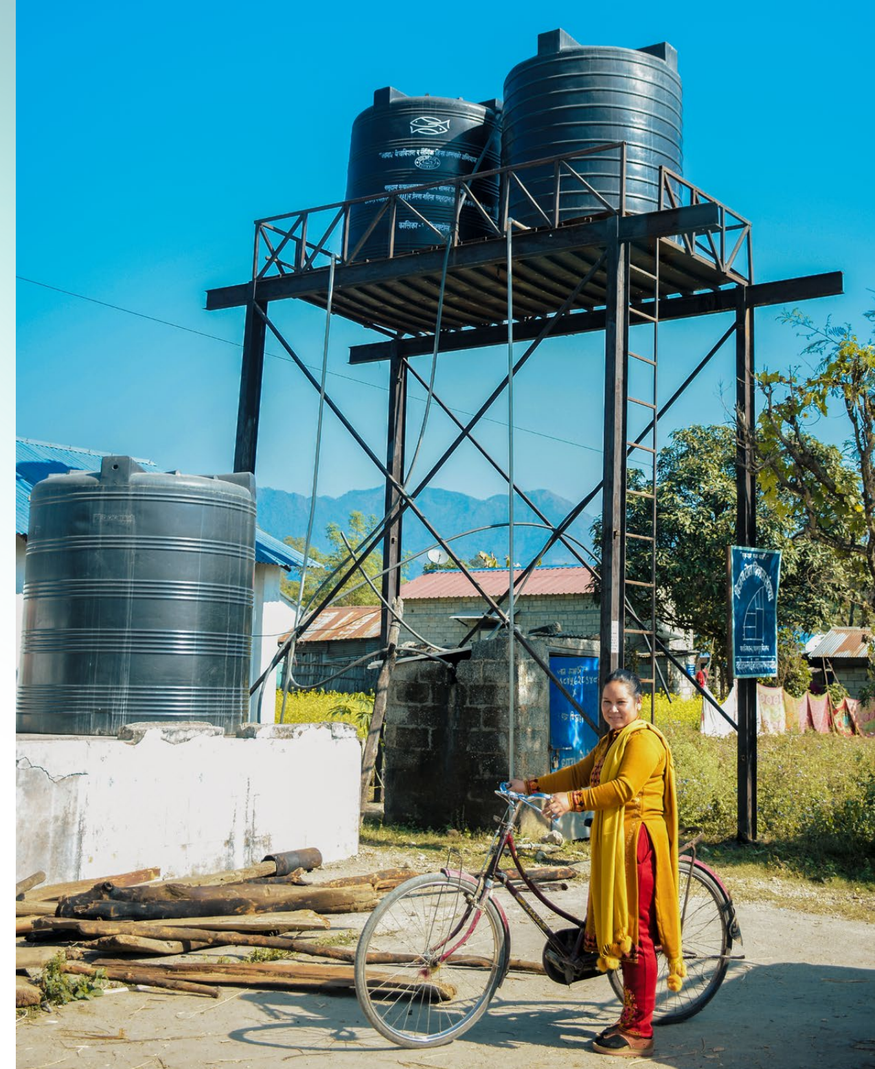
Pratima in front of the water supply tanks built in her home village.
