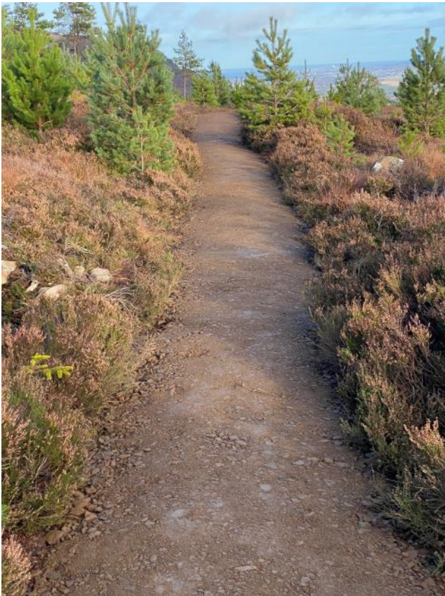
The repaired trail at Abriachan
