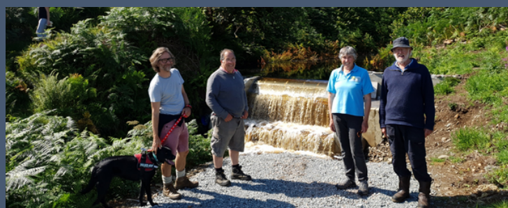
Sleat's community owned hydro scheme up and running
