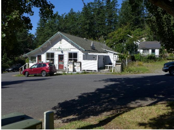
Fig. 1: East façade and vacant lot to the North
