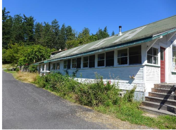
Fig. 2: South façade, entrance to apartment.
