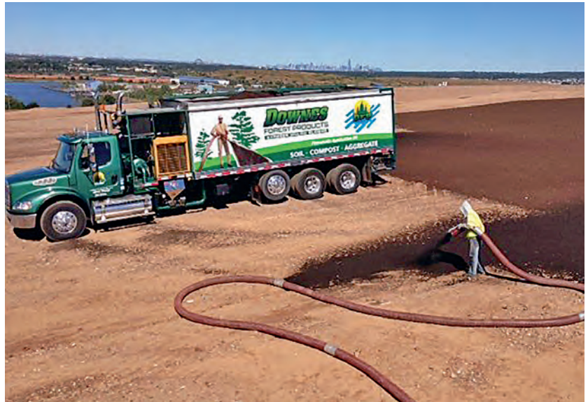
Applying compost mixed with plant seeds to control erosion at Freshkills Park in Staten Island.
