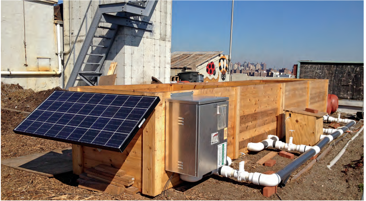
Solar powered forced aeration system in wood bins built by the NYC Compost Project Hosted by Big Reuse at Brooklyn Grange's rooftop farm in Long Island City.
