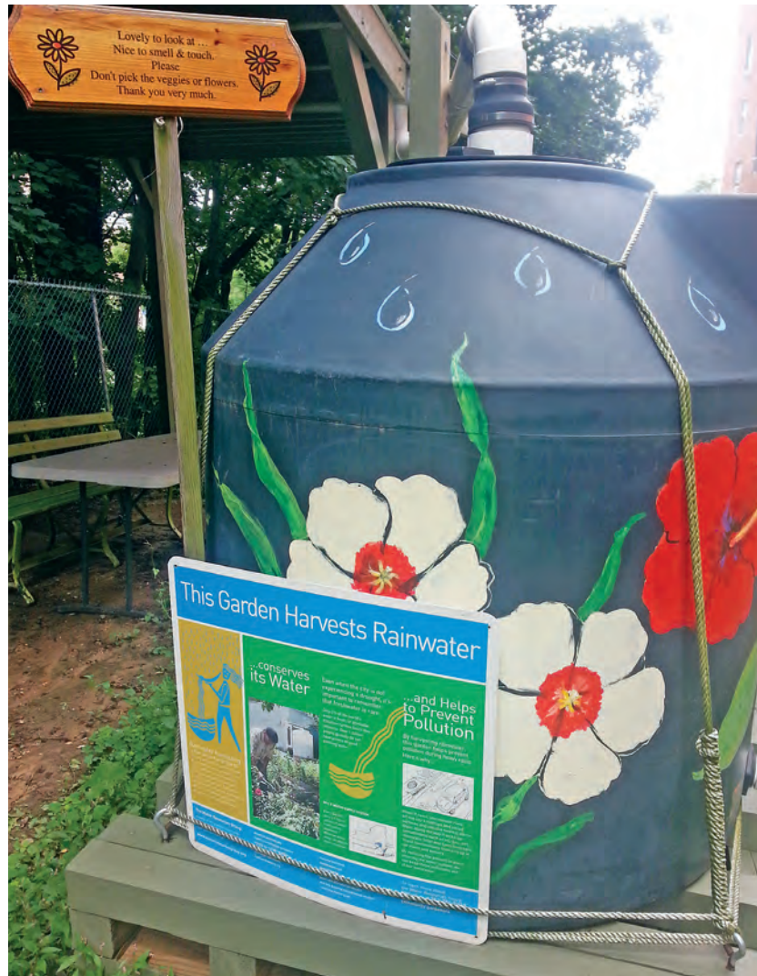
Rainwater harvesting system at Schervier Community Garden in the Bronx.
