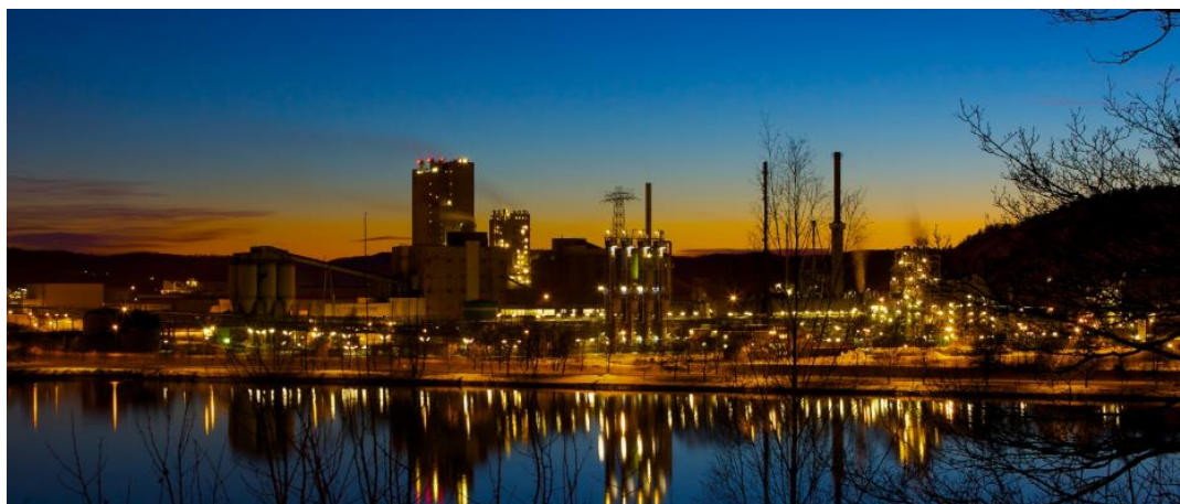
Figure 1-3 Yara ammonia plant at Herøya in Porsgrunn, Norway, is among the larger ammonia plants in the world (photo Ernst Vikne/Wikipedia). They have announced plans to start production of green ammonia.
