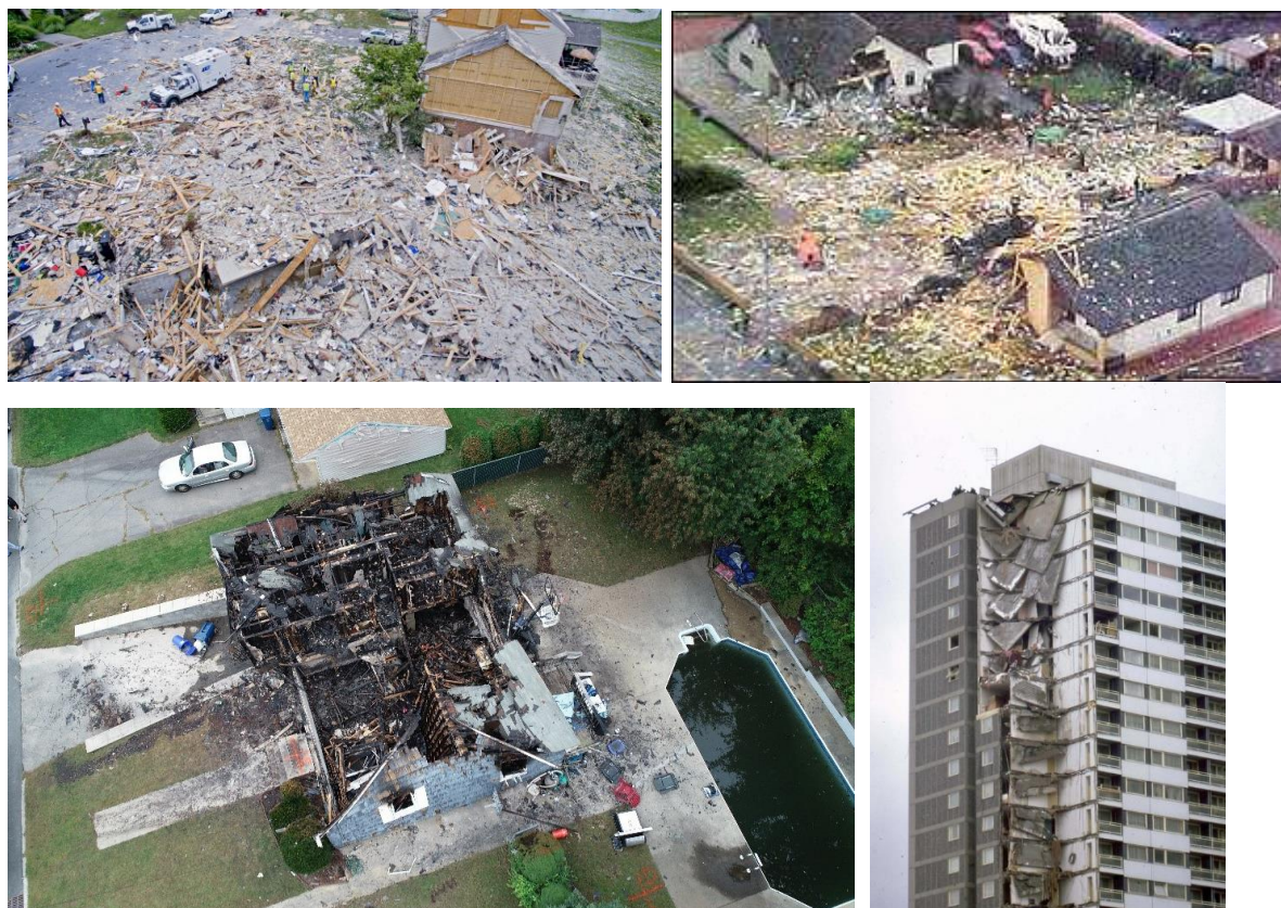
Figure 2-5 House explosions from Pennsylvania 2017 (Lancaster Online, upper left), from 1999 in Scotland (BBC, upper right), from Massachusetts 2018 (NTSB, lower left) and Ronan Point, England 1968 (Derek Voller, lower right)
