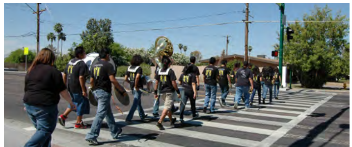
Ladder style high visibility crosswalk. Source: www.bikepedimages.org/Mike Cynecki
