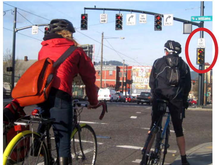
Bicycle signal head can be seen highlighted in the red circle. Source: National Association of City Transportation Officials
