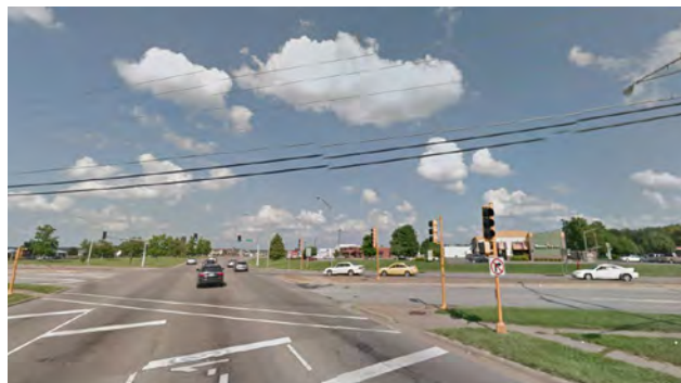
Existing Lewis Lane intersection: There is a lack of a crosswalk. A crosswalk should be added to connect to the multi-use trail constructed in 2015 on the west side of Lewis Lane.
