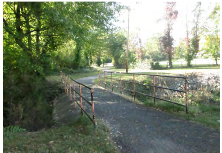
Greenway Bikeway: Existing bridge railings do not meet current standards and should be upgraded.
