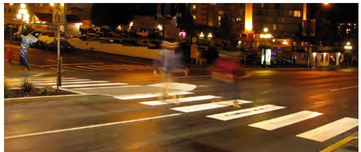
High visibility crosswalks are easier to see at night. Source: www.bikepedimages.org/Dan Burden
