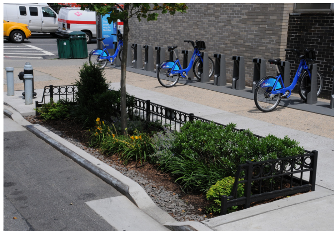
Bioswale (Credit: NYC Water)
