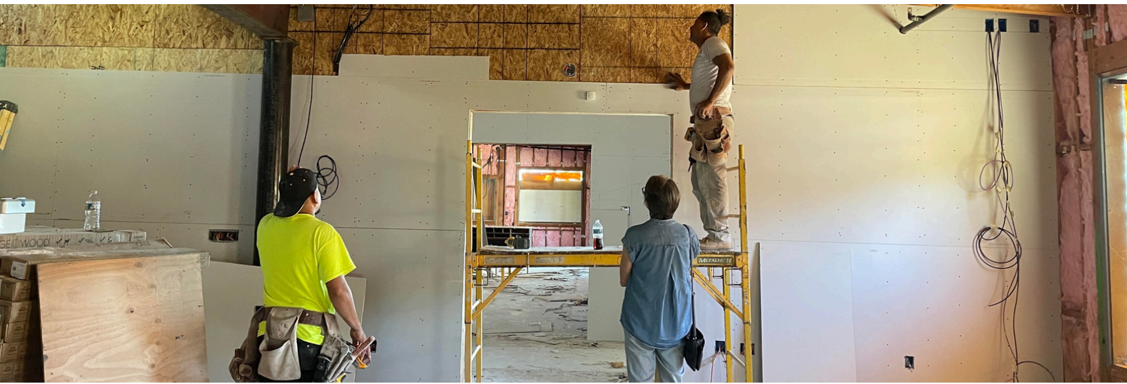
Insulation and sheetrock in the Gathering Space and Cafe.
