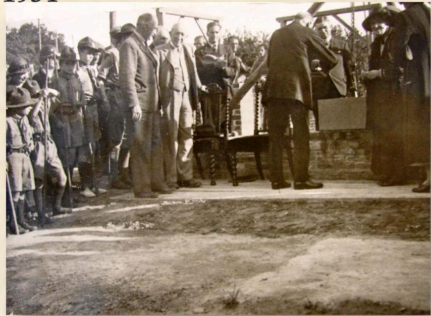
The stone being laid
