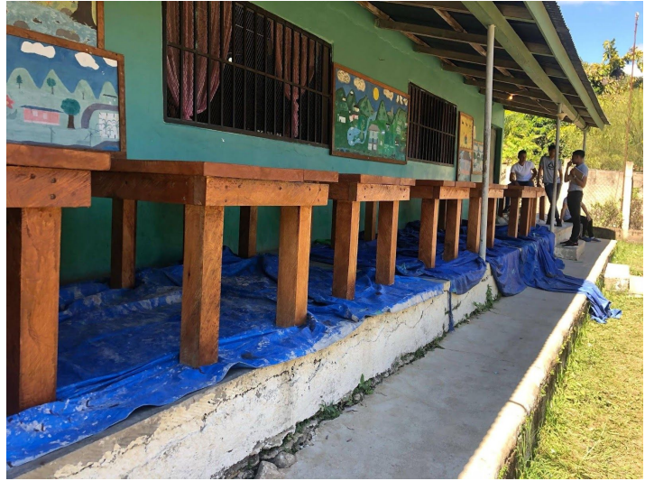
The completed tables lined up for one last inspection.
