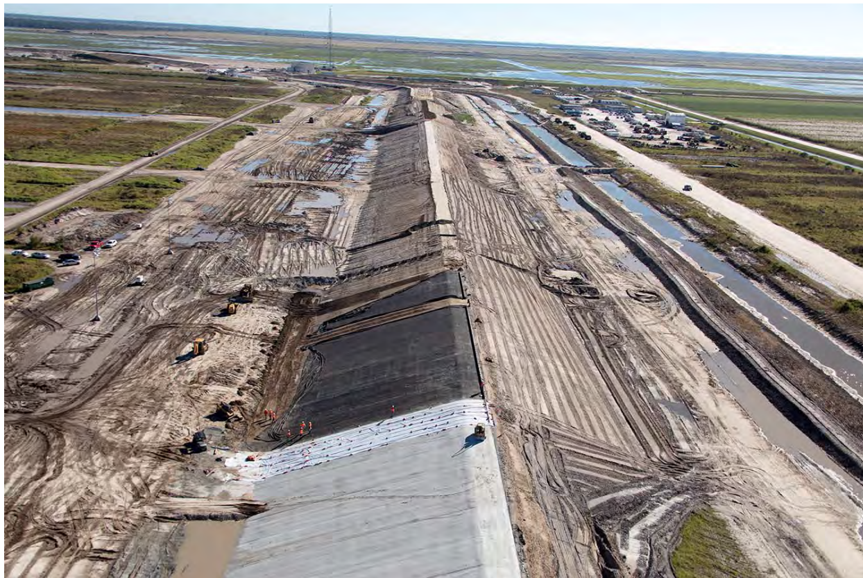
Aerial photo of C-44 Reservoir Embankment facing east (February 2020).
