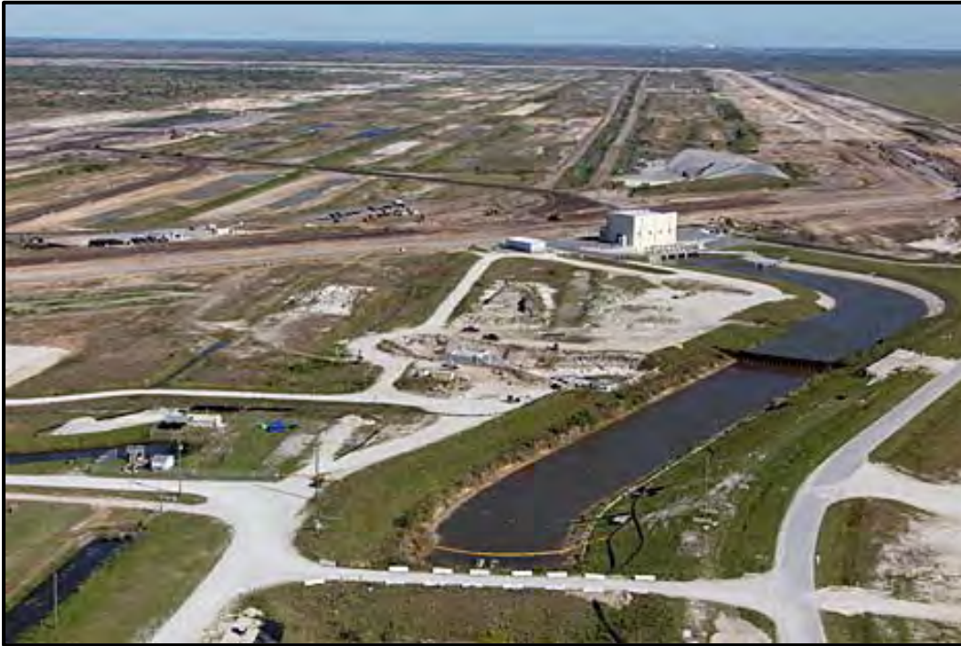
A view of the eastern embankment construction of the C-44 Reservoir.
