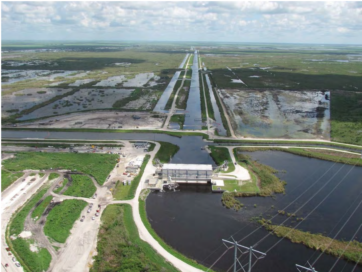
Re-configuration of STA 1W outflow canal at G-310 pump station.
