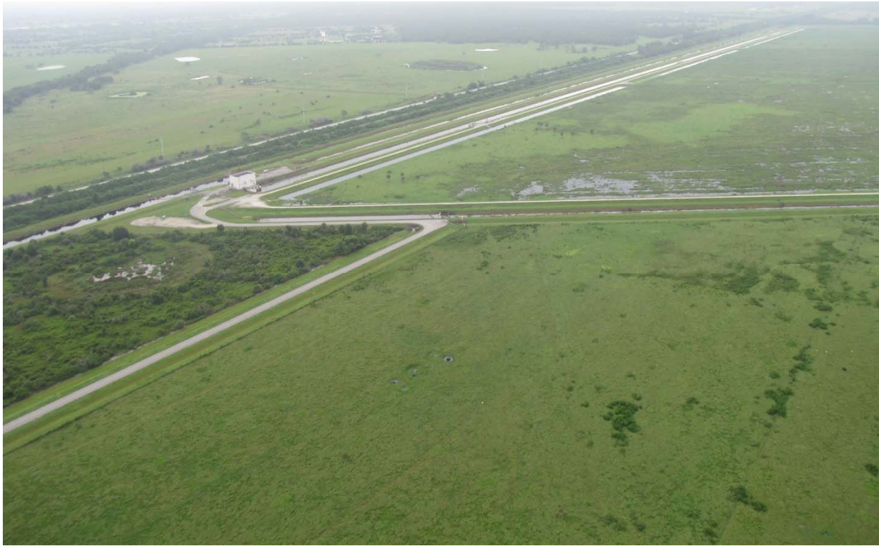
Lakeside Ranch Phase I – Northern STA and S-650 Pump Station
