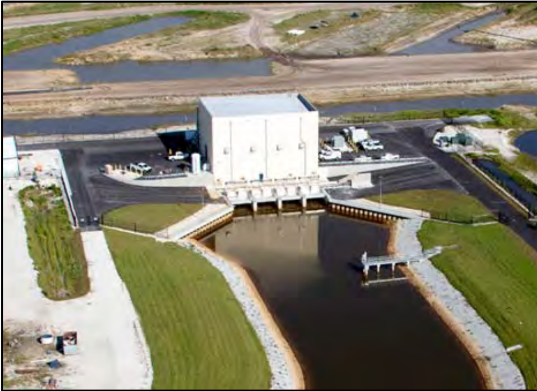
Southern view of the completed C-44 Pump Station.
