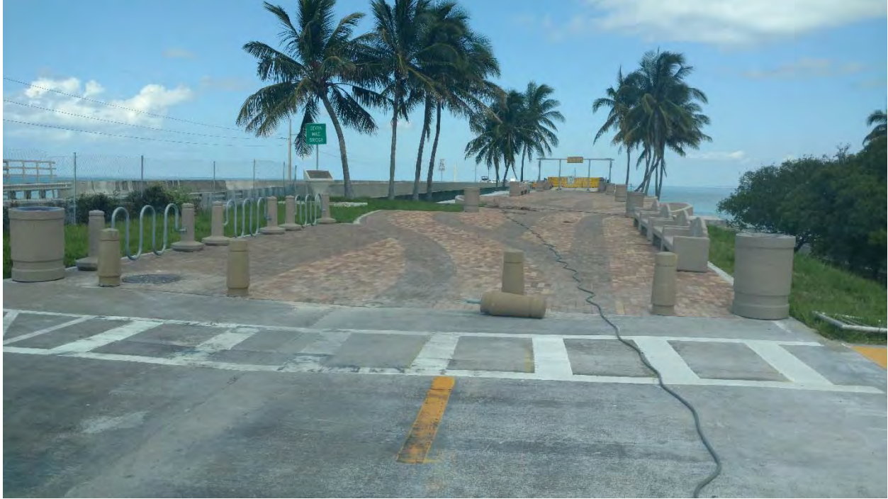
Knight's Key Old 7 Approach (Currently FDOT Contractor staging area).
