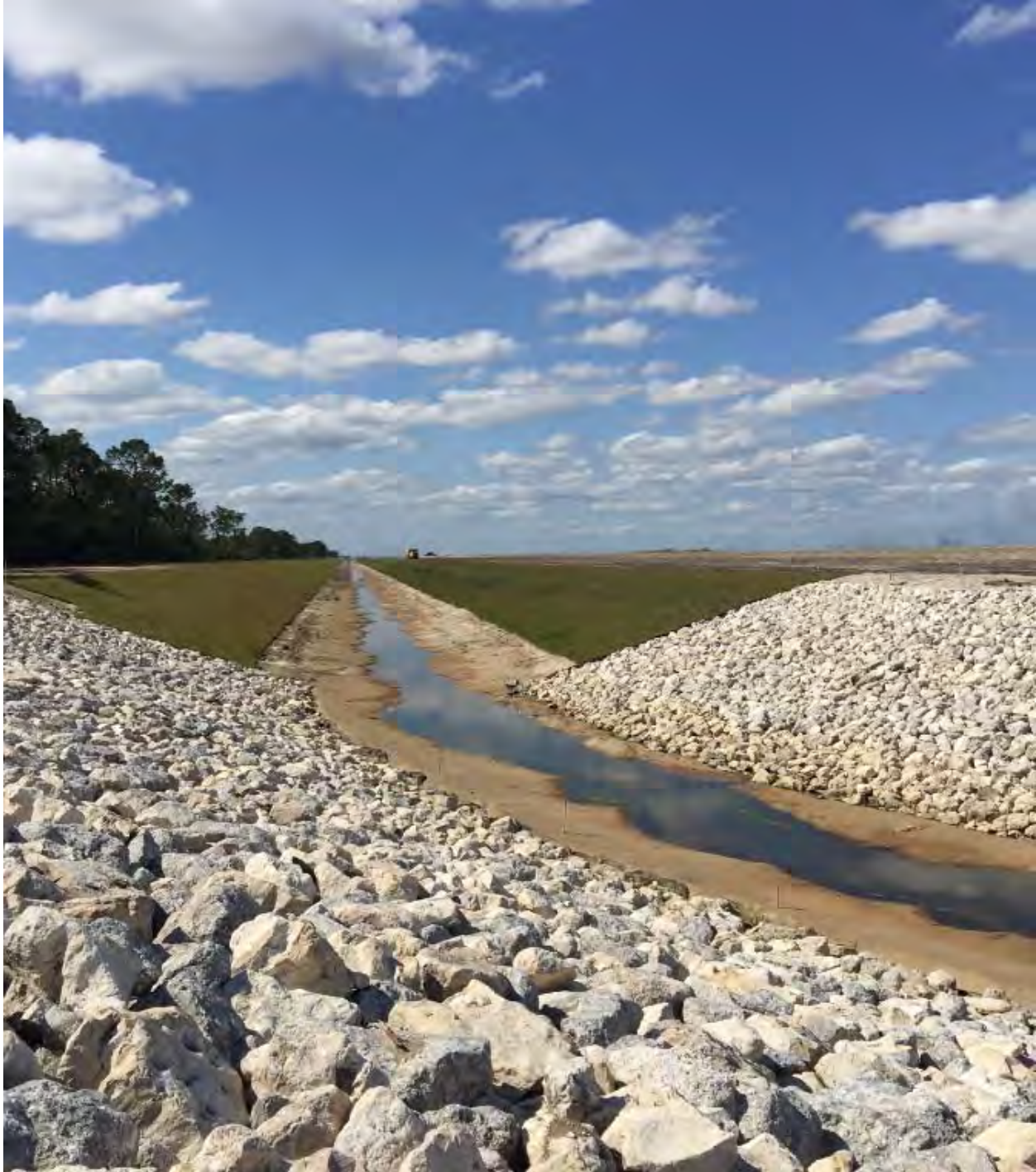
Southern view of the C-44 STA southbound collection canal from the north east corner of Cell 2.
