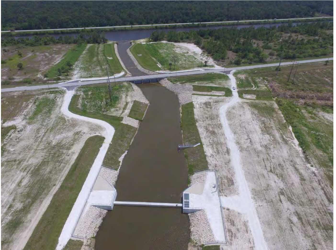
Southern view of the C-44 STA discharge canal, the C-44 System Discharge Structure S-404, and the C-44 Canal.
