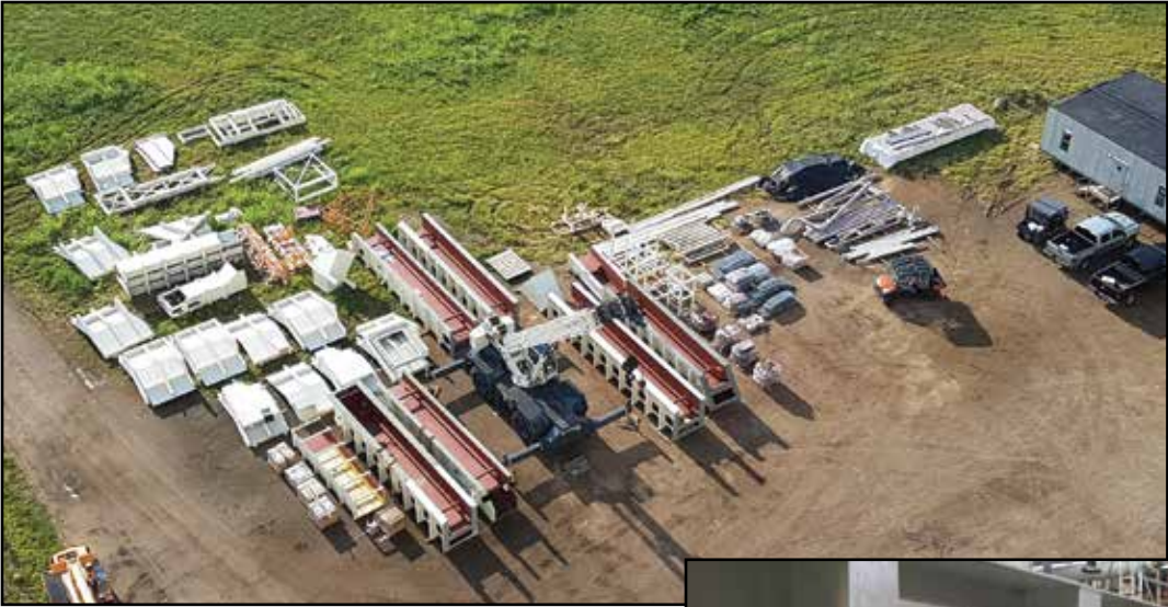
Conveyor sections await installation during the planned Hugo Plant maintenance outage.
