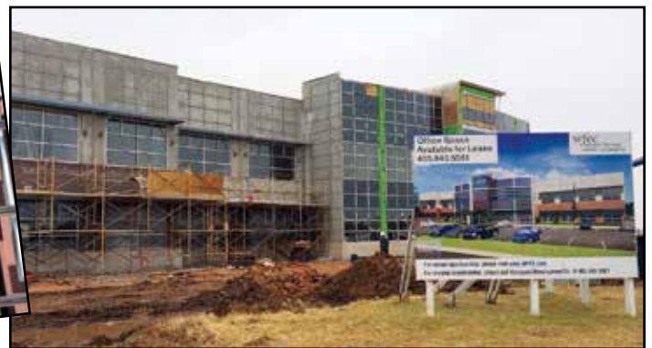
Walls going up and nearing completion at new Moore Office site.
