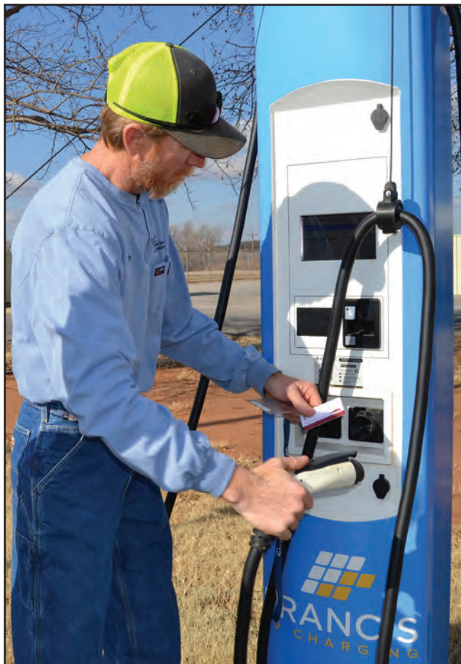
Kevin Orrell prepares to use an RFID (radio frequency identification) card in order to charge one of WFEC's electric vehicles from the company fleet. Level 2 chargers are located at WFEC's facilities.
