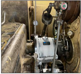
During the existing outage currently being performed on Anadarko Units 5 & 6, a newer style of clutch assembly was installed. Previously, the original, old style clutch/jaw assembly was utilized. These were recently replaced with a Synchronous-Self-Shifting (SSS) clutch assembly that promises higher reliability during startup and shutdown, plus fewer maintenance issues.
