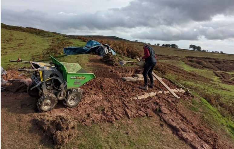
Plate 12 - Scrape 5 during repair, looking south
