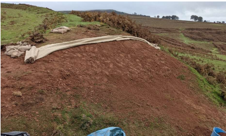
Plate 13 - Scrape 5 after filling, looking south. Hessian was placed over the repairs.
