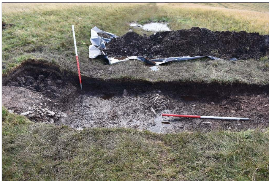
Plate 15: Excavated features in the east end of Trench 1, looking south
