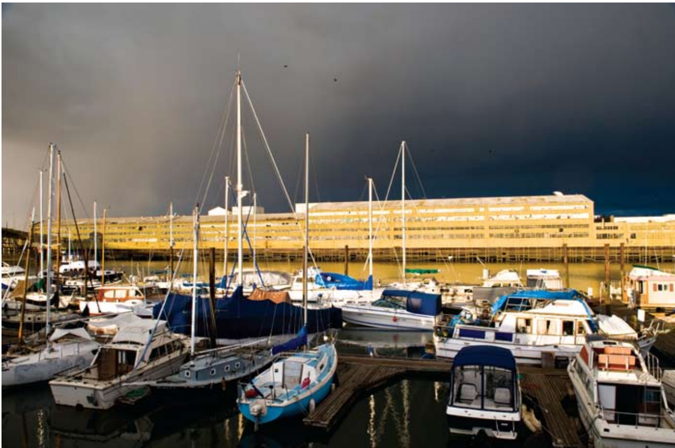
The Boeing Company's Plant 2 – now nearly empty –sits across the river from the South Park Marina
