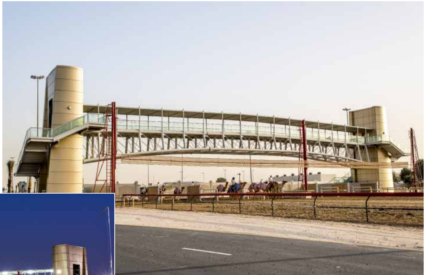
Camel Race Track Footbridge, designed and built by Waagner Biro Gulf LLC in 2013.
