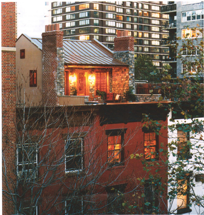
With its copper roof, double chimneys and hand-carved porch furniture, the cabin is an idyllic rural retreat in the heart of Manhattan.
