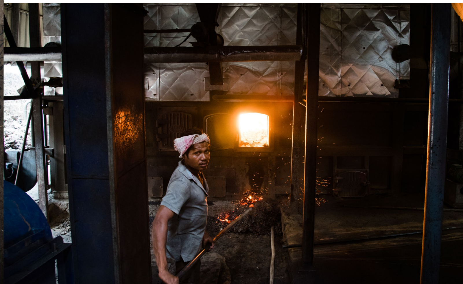
Worker operating boiler at fishmeal and oil company at Ullal, India
