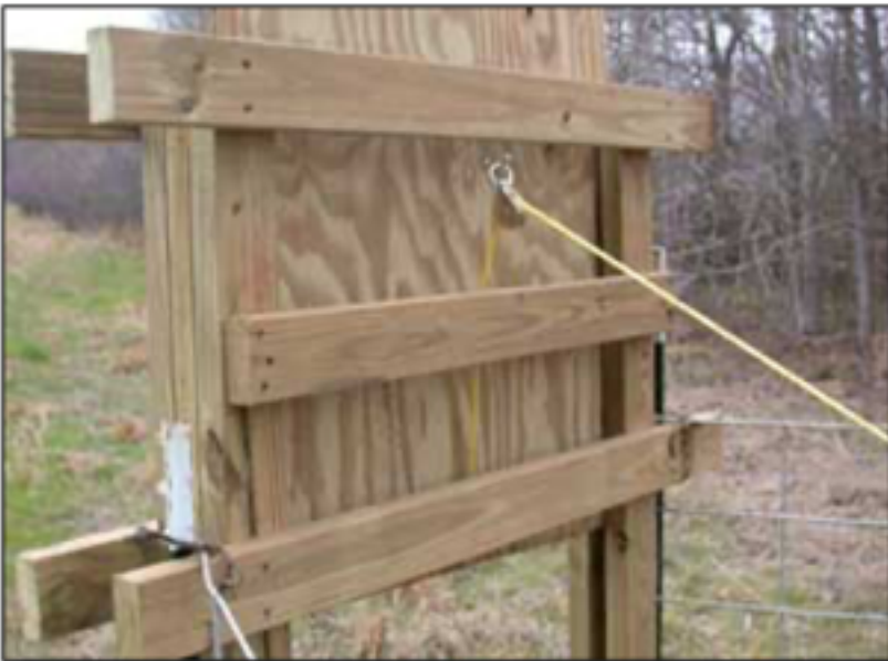
Figure 2.18. A wooden guillotine door. Notice the rope guided through the pulley; this stops the rope from hanging up when closing.
