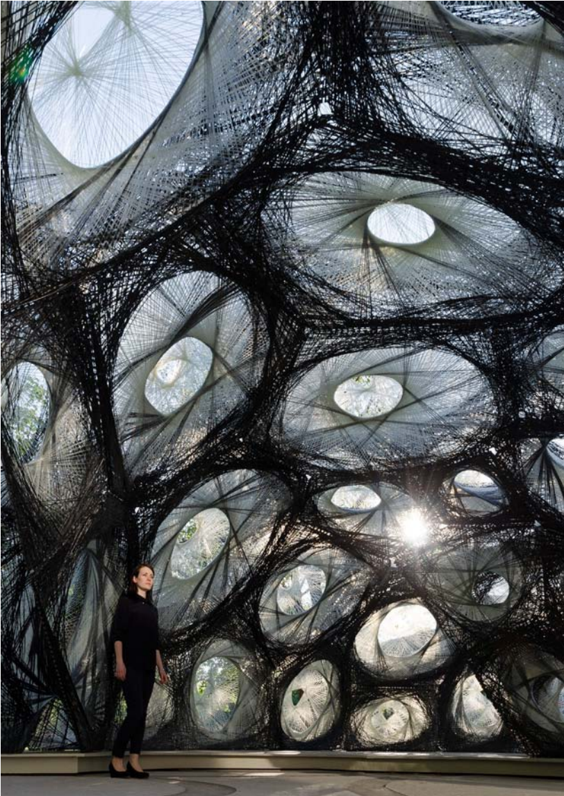
Figure 13. Thirty-six unique components were generated for the lightweight pavilion. © ICD/ITKE University of Stuttgart.
