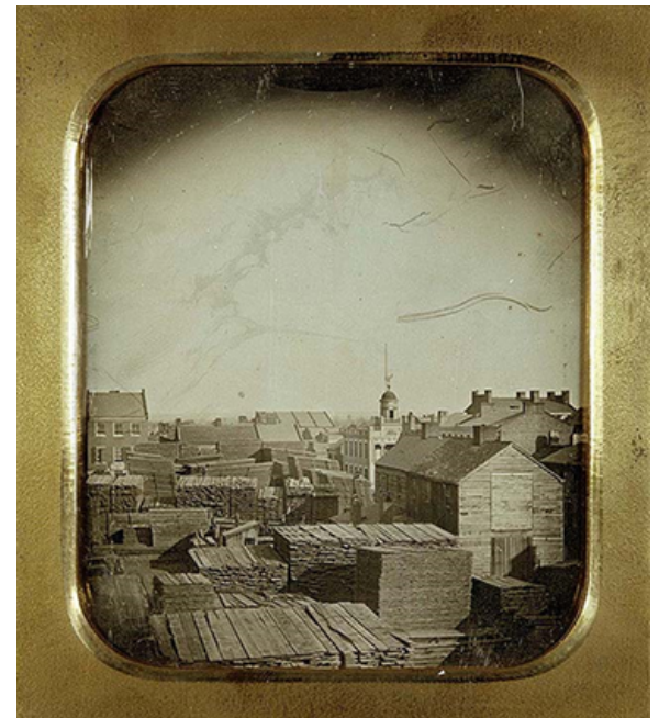
LOCUST STREET LOOKING EAST FROM FOURTH
