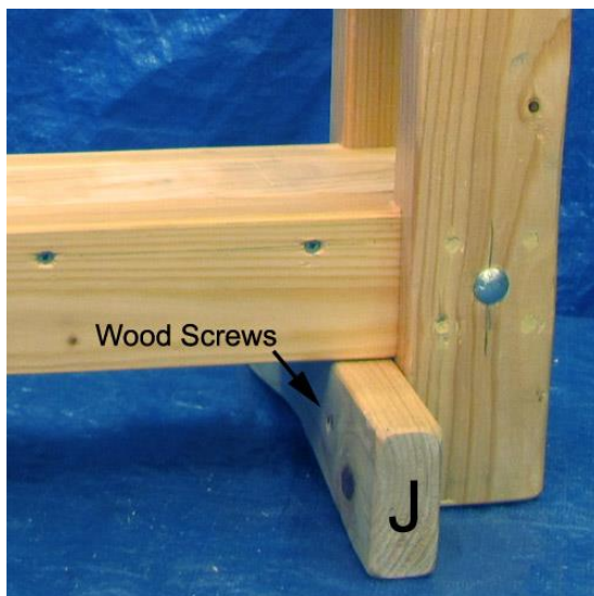
15. Attach J using 2 1/2" wood screws or 3" nails
