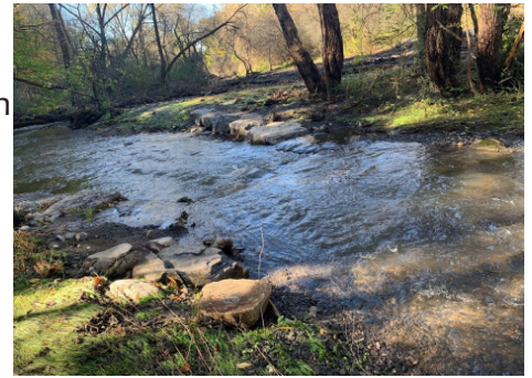
Shotwell Brook stream restoration project in the Town of Skaneateles
