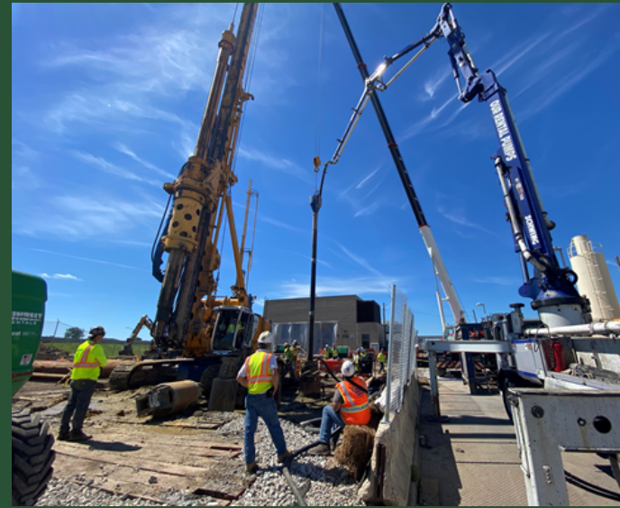
Crews install Secant Piles at Bay Park Shaft 1
