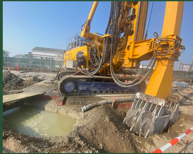
CSM being performed at Bay Park Shaft 2
