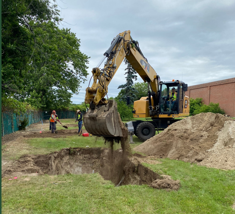
Crews performing test pits at Cedar Creek Shaft 3
