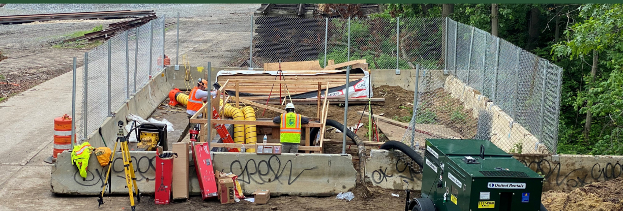
Crews inspect the existing Sunrise Highway aqueduct at Pit P
