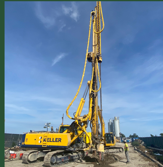
SOE is set at Bay Park Shaft 2 (Photo: August 2021)
