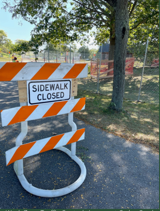
Work Zone Traffic Control signage at Cedar Creek Shaft 3 (October 2021)
