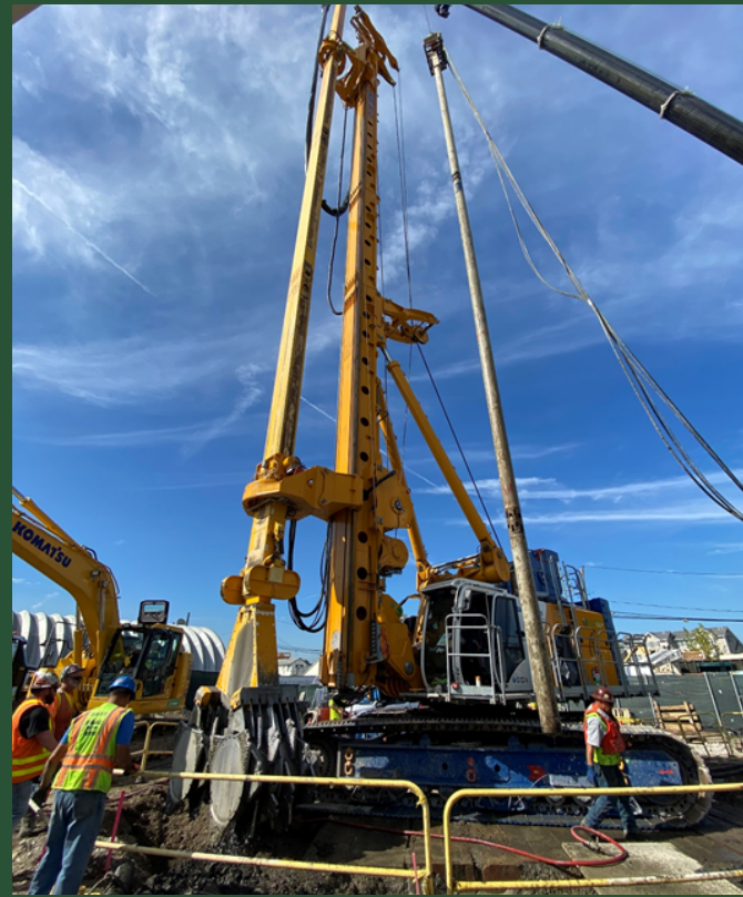
SOE being installed at Bay Park Shaft 3 (October 2021)
