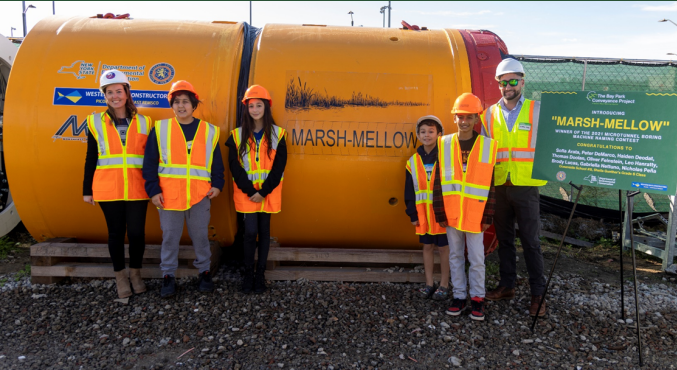
MTBM named MARSH-MELLOW at Bay Park Shaft 2 (November 2021)
