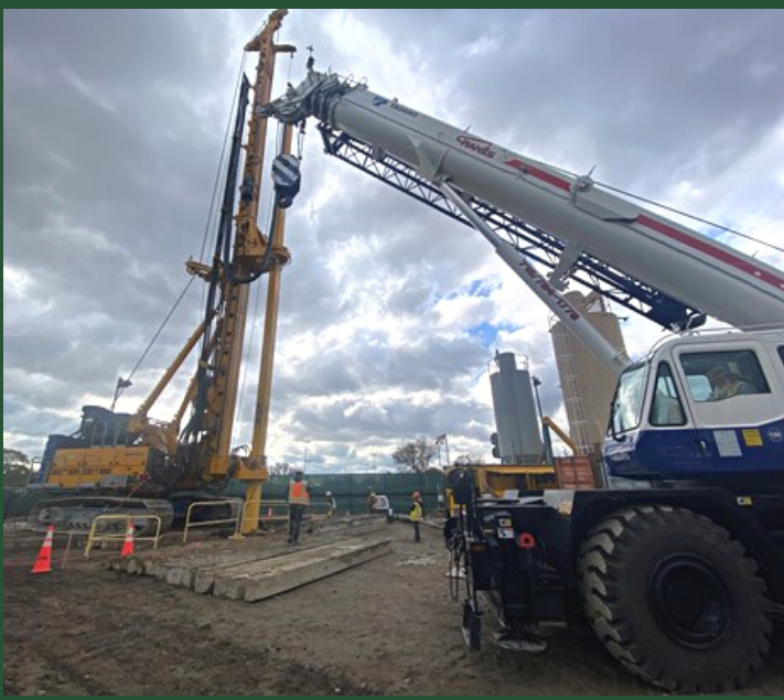
Installation of CSM Panels at Bay Park Shaft 8 (November 2021)
