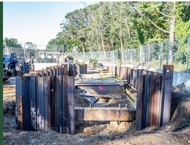
Construction at Pit P along the Sunrise Highway Alignment (October 2021)
