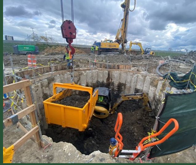
Shaft excavation at Bay Park Shaft 1 (November 2021)
