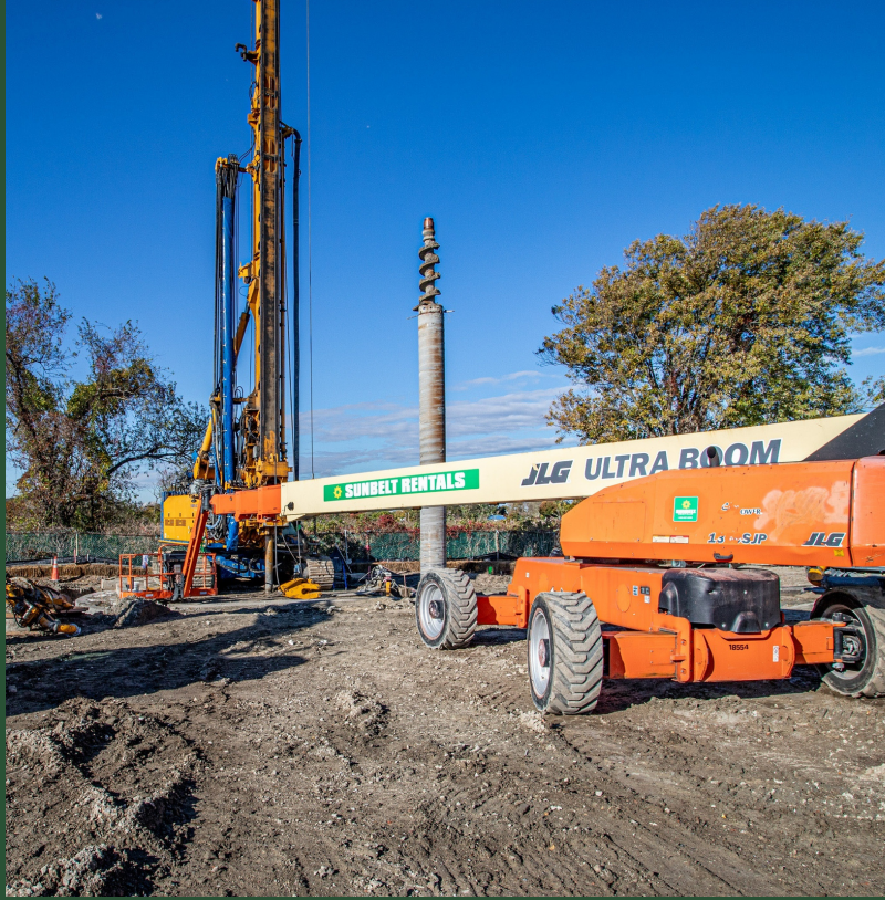
SOE installation at Cedar Creek Shaft 2 (November 2021)
