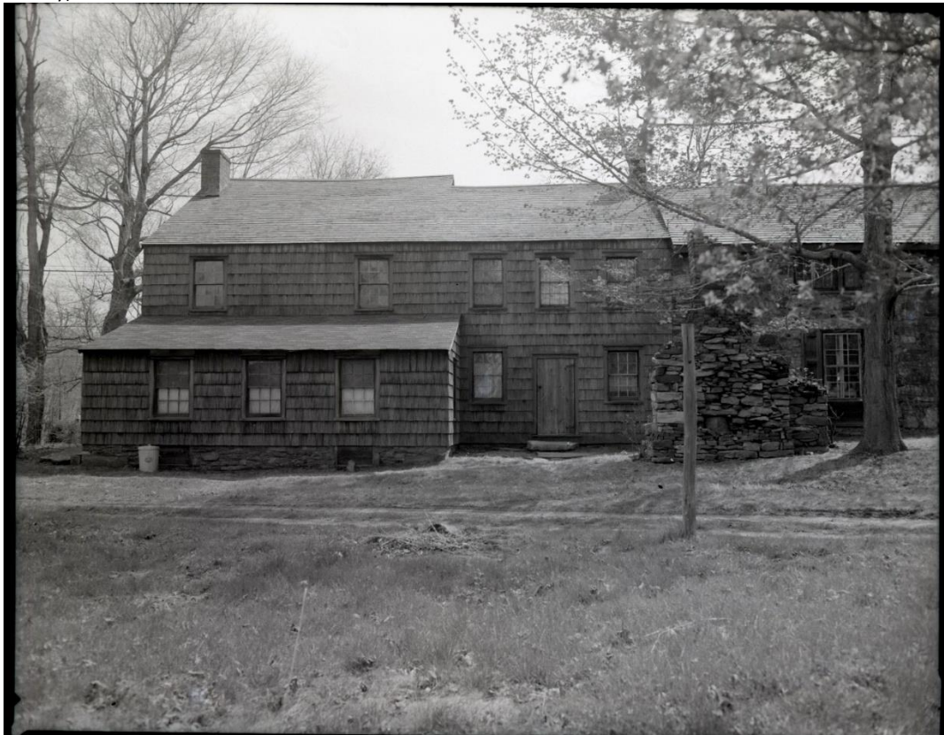
Figure 21. Undated photograph of the rear of the Odell house, likely in the 1970s (Westchester County Historical Society).
