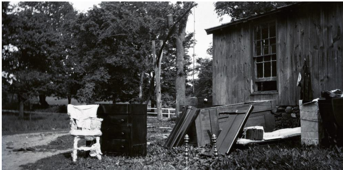
Figure 25. Historical photograph (circa 1920s) of the northern portion of the Odell House with the well just hidden from the photo. A well sweep is seen, with two large branches utilized as levers to retrieve water from the well (Westchester County Historical Society).
