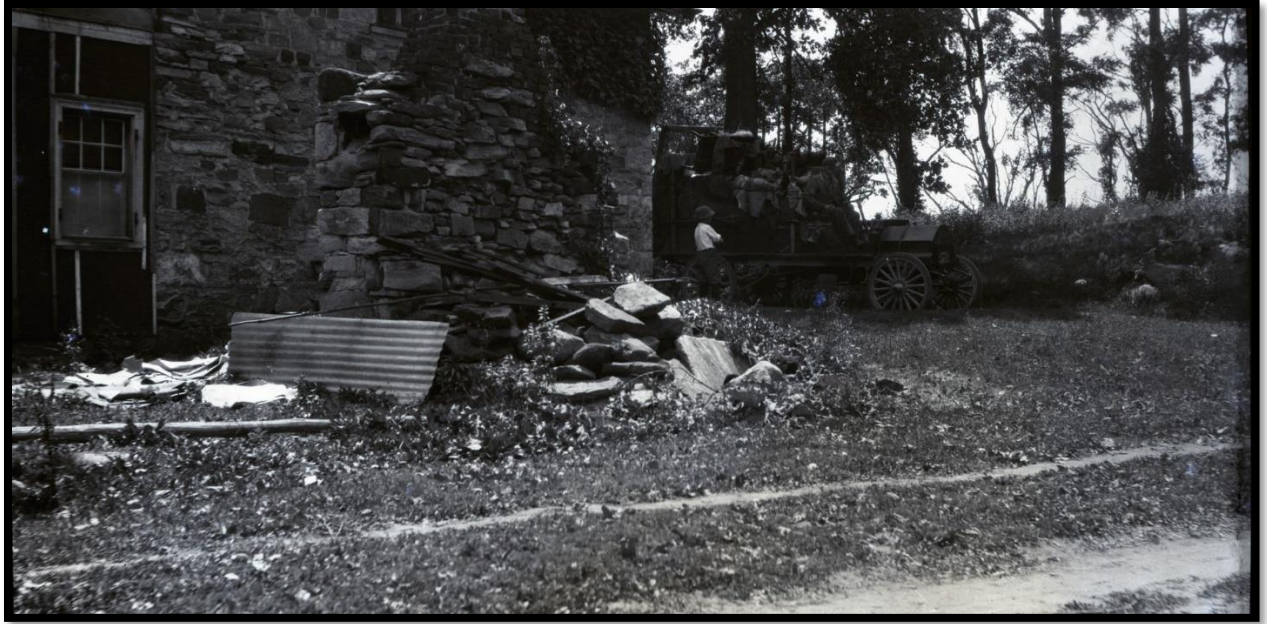
Figure 18. The rear of the house in the 1920s, this view shows the detached chimney had along been abandoned and partially dismantled by this time (Westchester County Historical Society).
