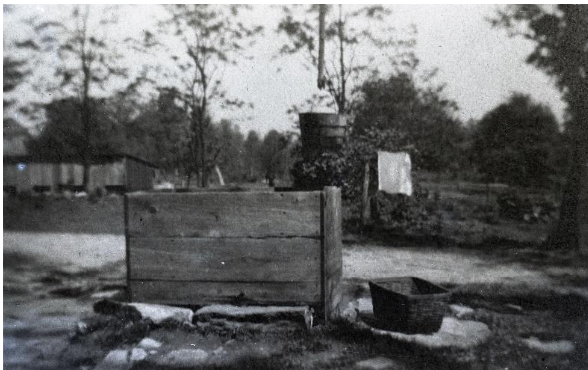
Figure 26. A detailed view of the well with its stone lining, wooden box walls and bucket attached to a well sweep, circa 1920 (Westchester County Historical Society).
