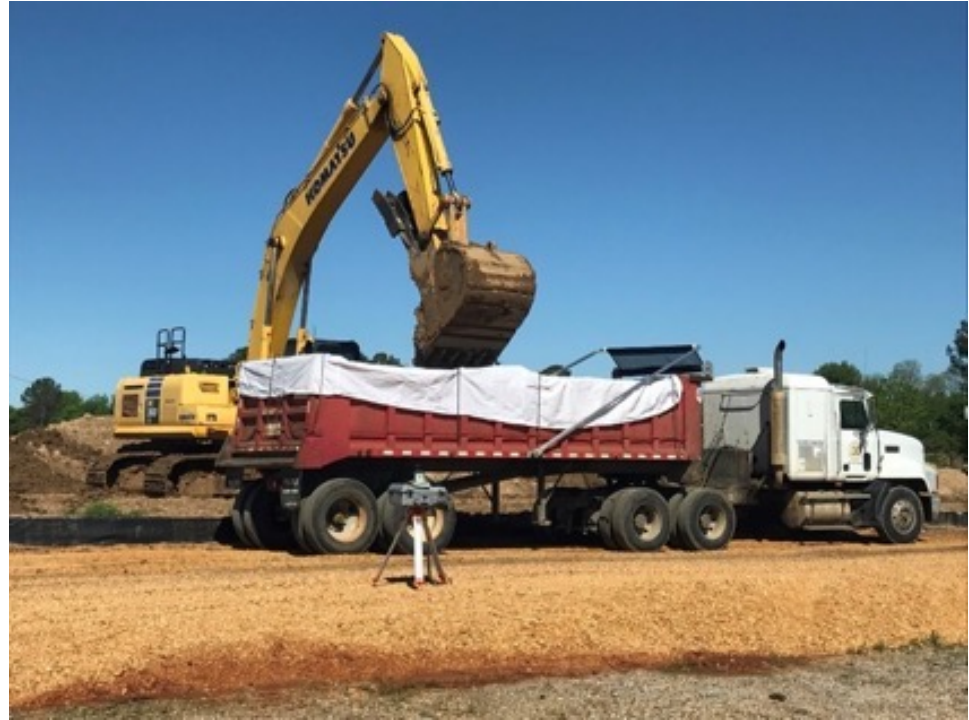
Photograph of Excavation Remedial Action at Kerr-McGee Columbus, MS Site
