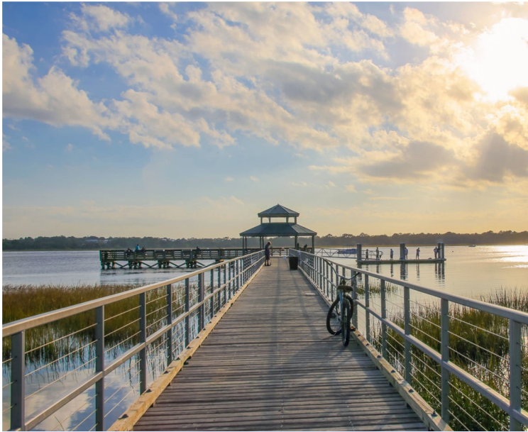
Example Image: Fixed Pier with Gazebo
