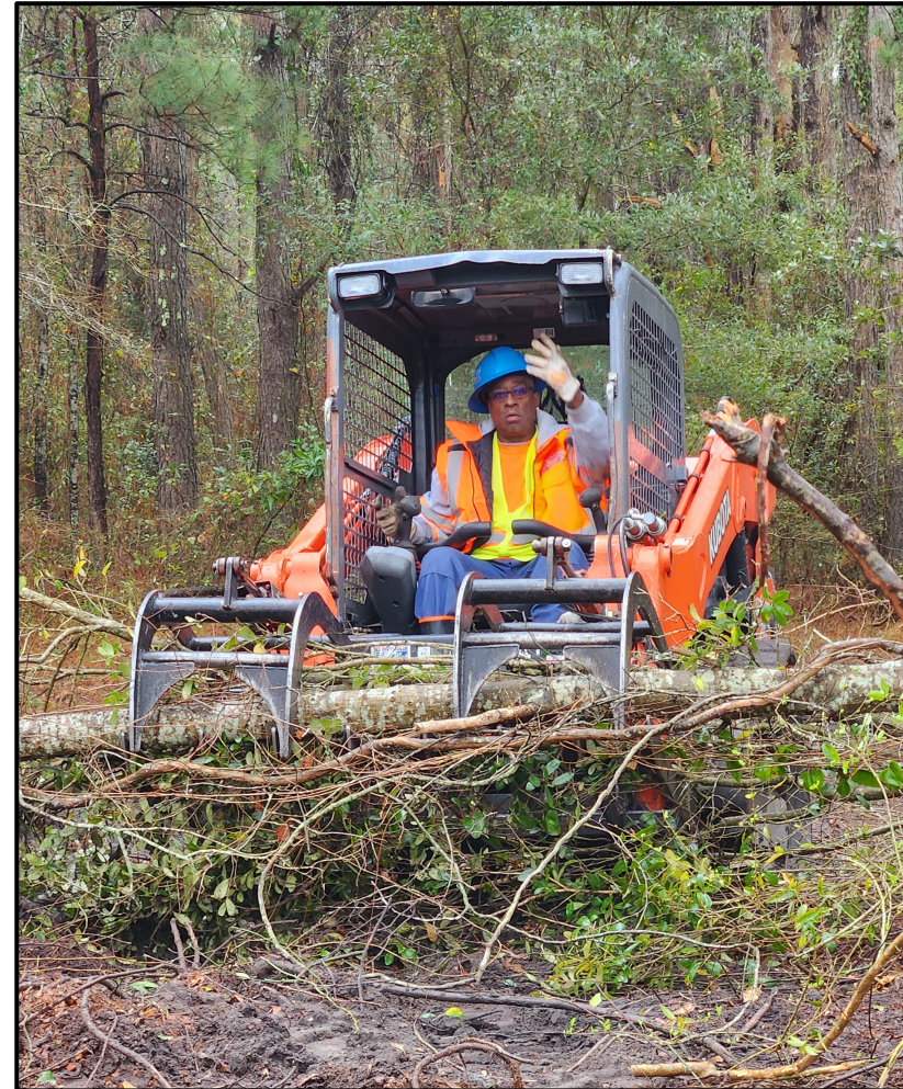
Worker performing vegetation clearing
