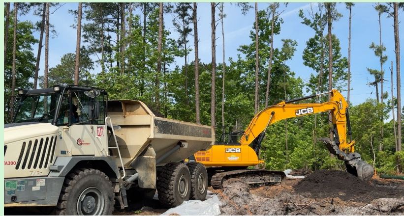
Contractors loading excavated soil in OU2 for transport to stockpile in OU4
