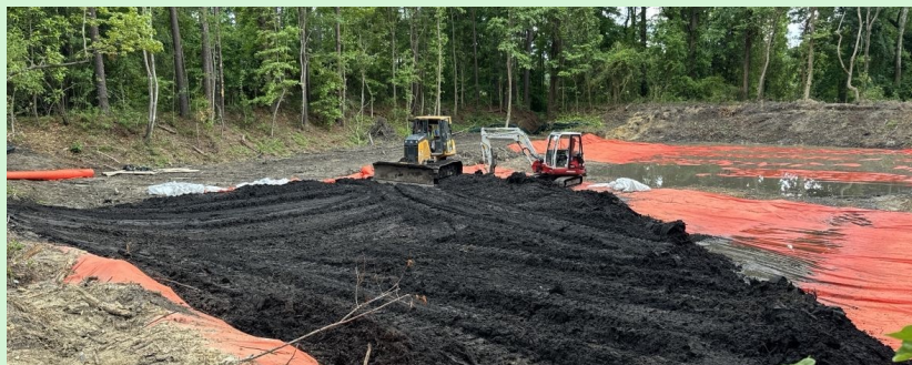
Contractors spreading excavated OU2 soils in former fire pond stockpile in OU4
